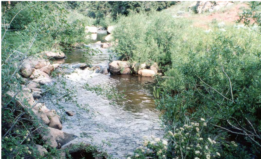
Figure 30-6. The same view seen in Figure 30-5 11 years after the structures were built. Riparian vegetation has responded positively to reduced cattle grazing, sediment deposition, and improved subirrigation of the riparian zone near the plunges.
