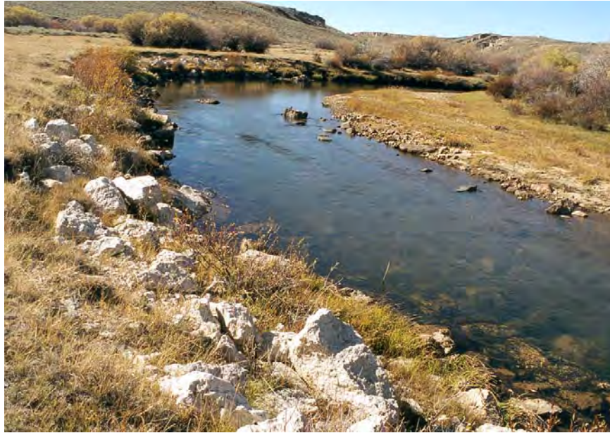
Figure 62-3. A formerly eroding bank as it appeared 25 years after it was stabilized with limestone chunks. Willows have become established along the bank behind the riprap to further stabilize it. Compared to surrounding willow clumps, the new willow growth is still short, even after 25 years, which points out the long period of time sometimes necessary for riparian vegetation to become reestablished after severe disturbance.
