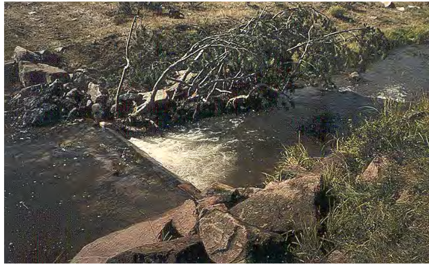
Figure 1. The WGF Aquatic Habitat Construction Crew did the installation of stream habitat improvement structures for most projects. Here they are building a timber plunge in Big Willow Creek (top photo) and the completed plunge, with its plunge pool and a cover tree along one side, is shown in the bottom photo.
