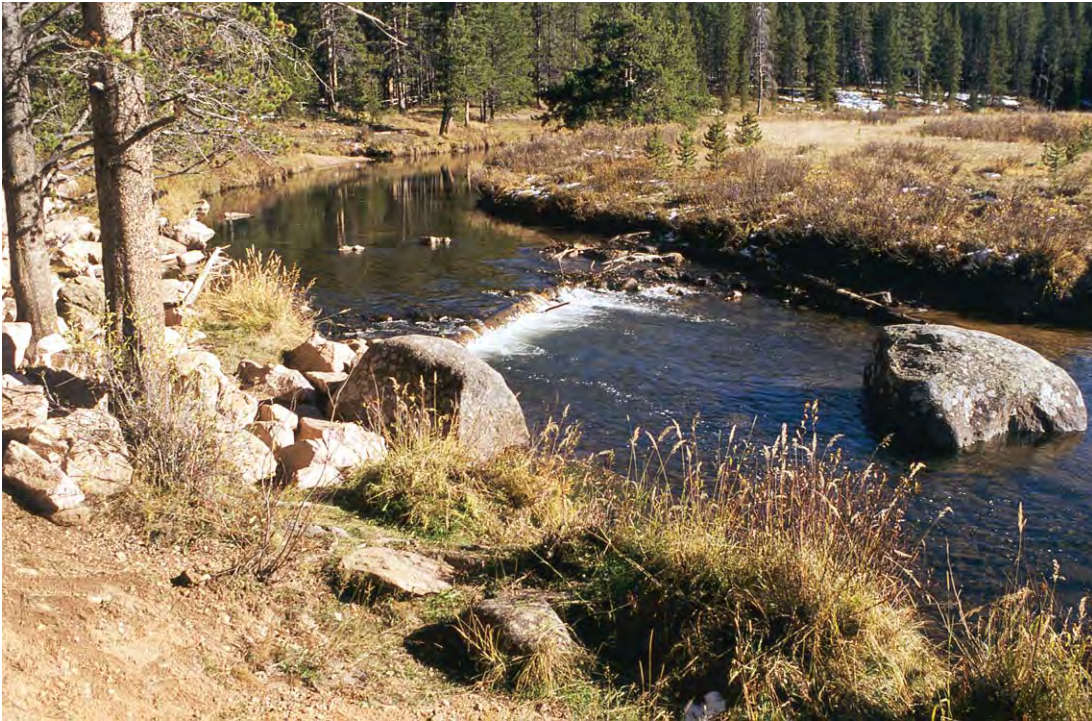
Figure 57-3. A diagonal digger log weir was built to provide deep pool habitat in a shallow run.
