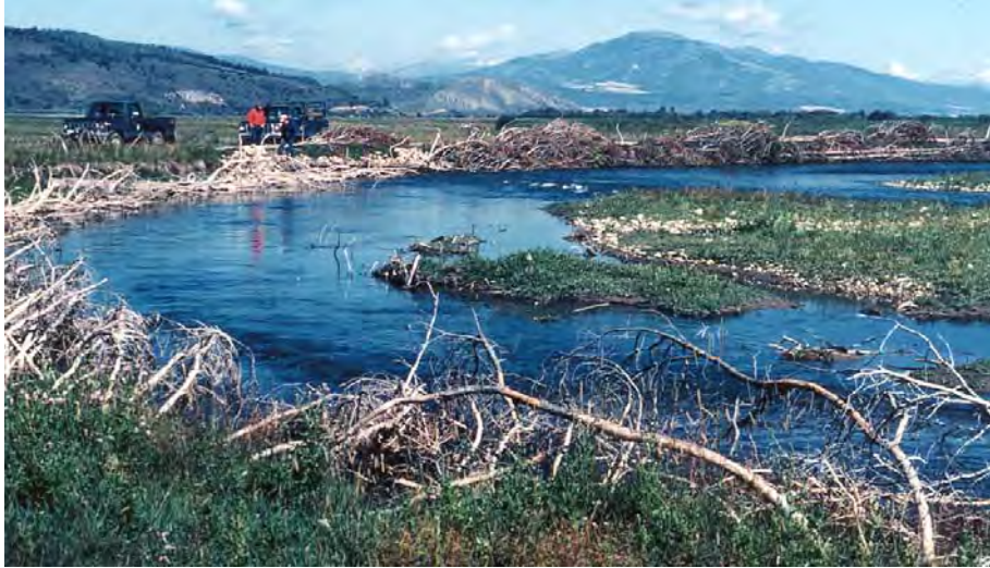
Figure 54-1. Tree revetments were installed in the Salt River to protect eroding banks.
