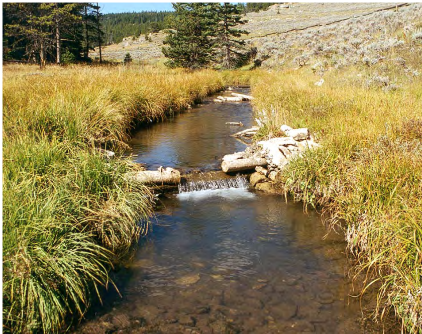
Figure 18-2. This log plunge in a meadow section of Fool Creek is intact and providing pool shelter for trout 19 years after being built.
