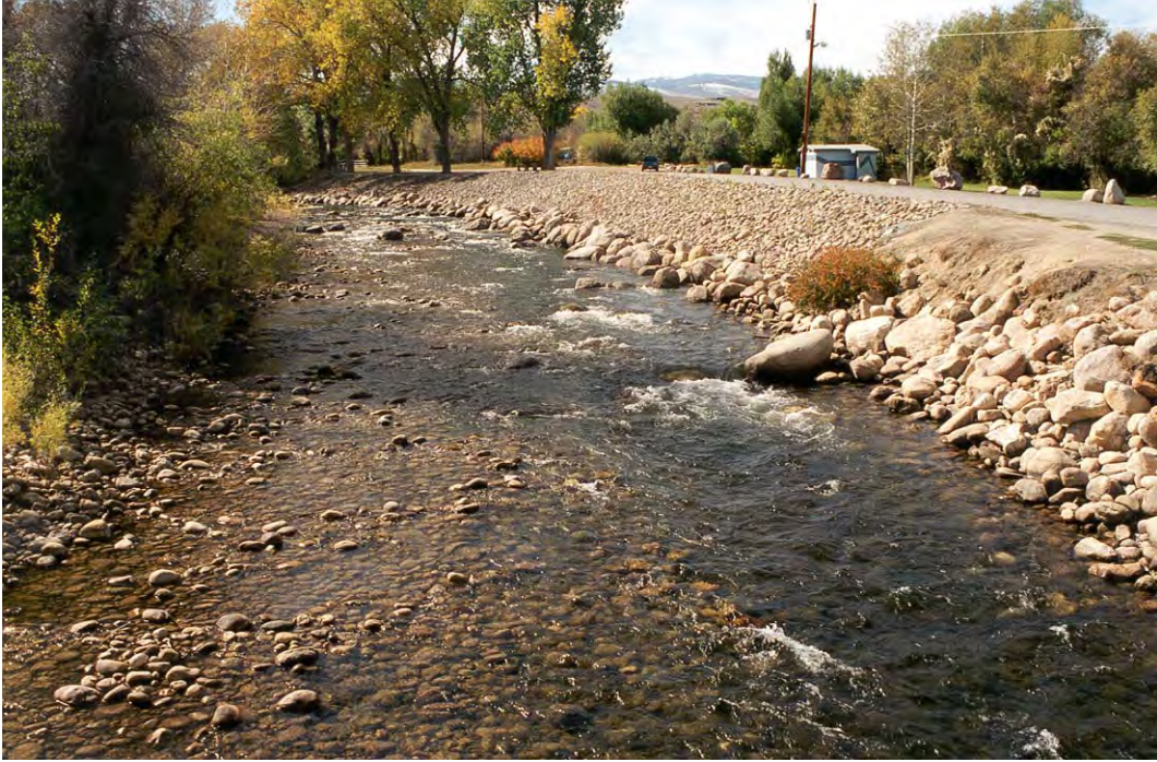
Figure 38-2. Pretreatment, low flows in the Middle Fork were spread shallowly across the riverbed due to previous channelization. Posttreatment, the river has formed a deeper thalweg near the right bank, thus concentrating low flows to aid trout.
