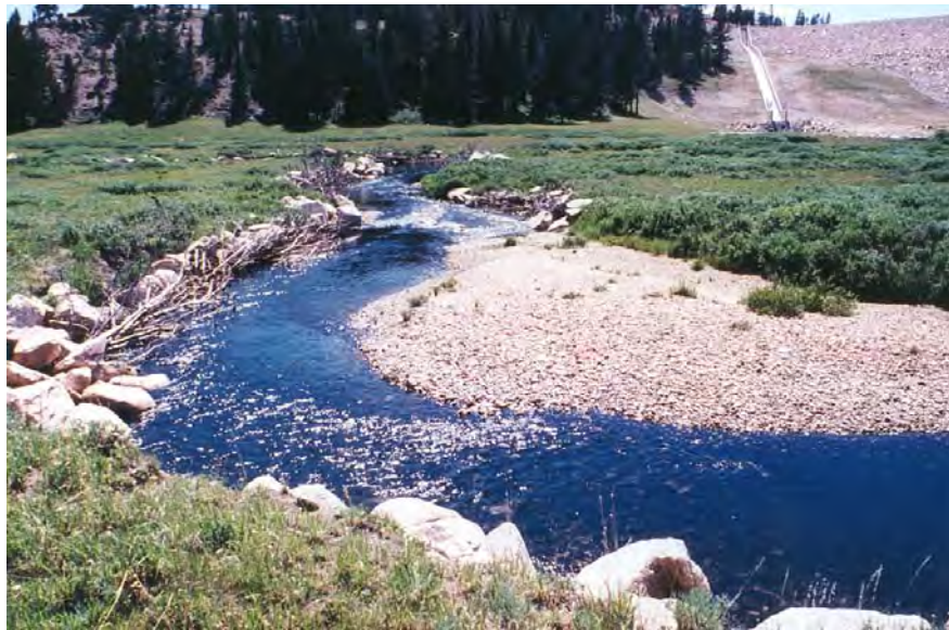
Figure 27-1. Stream banks scoured bare by flood waters were stabilized with tree and rock revetments, which narrowed Hog Park Creek and provided shelter for trout. This picture, taken three years posttreatment, shows riparian vegetation starting to establish on the point bar. By 1997, more vegetation had developed on the bar.
