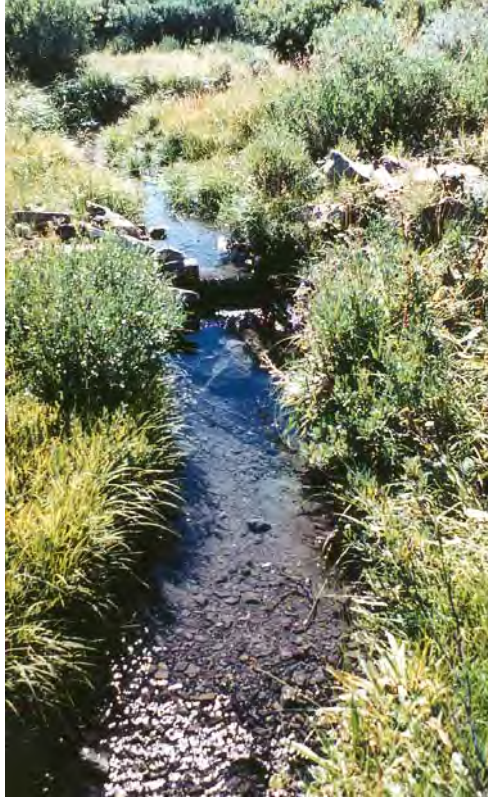
Figure 40-2. Timber plunges built in tiny Nameless Creek acted as grade controls and provided additional shelter for CRC trout.
