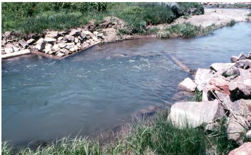
Figure 53-2. An upstream “V” log plunge (log vortex weir) produced a deep plunge pool that provided excellent shelter for trout in Salt Creek.
