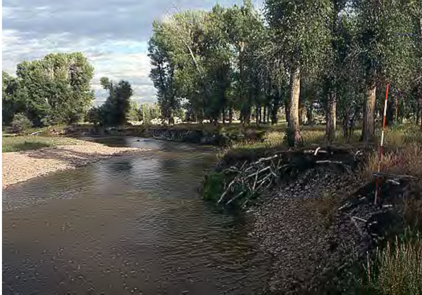
Figure 2-1. An eroding stream bank along the Bear River at the Bear River State Park before bank stabilization.
