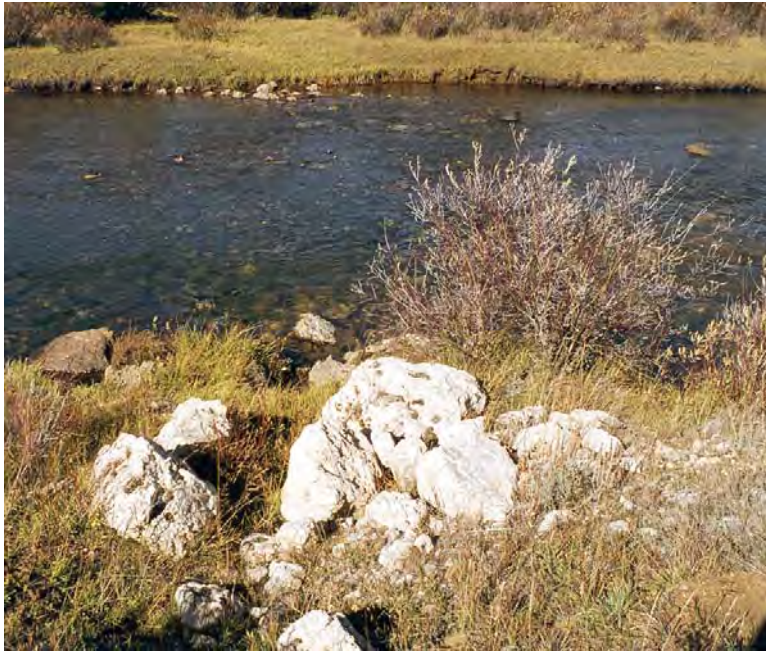
Figure 62-5. A few limestone boulders on the bank are all that remain of a rock weir after 25 years. The stream has presumably buried the instream portion of the weir.
