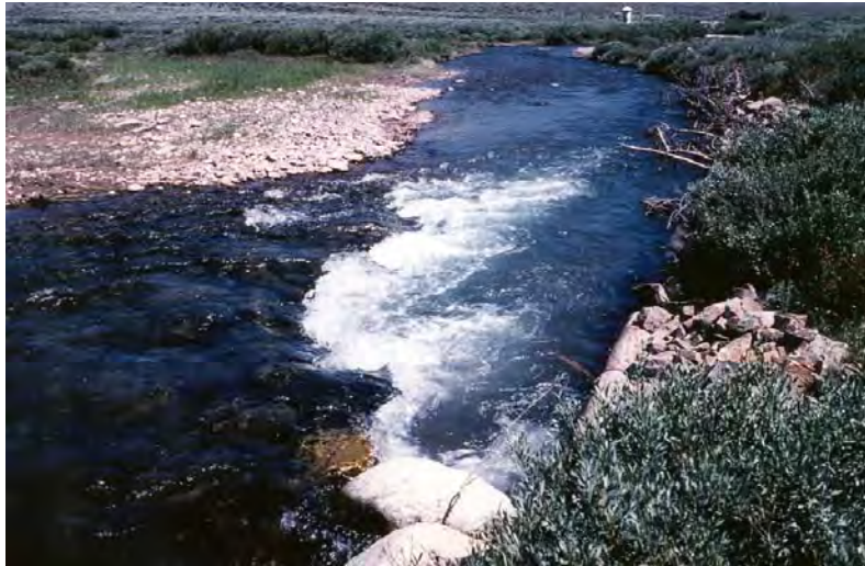
Figure 55-5. A diagonal rock weir was coupled with a tree/rock revetment to provide a deep pool having considerable woody debris shelter. Electrofishing always found many trout in this patch of cover. The weir extends from the large light colored rocks in the foreground across the stream into the point bar.
