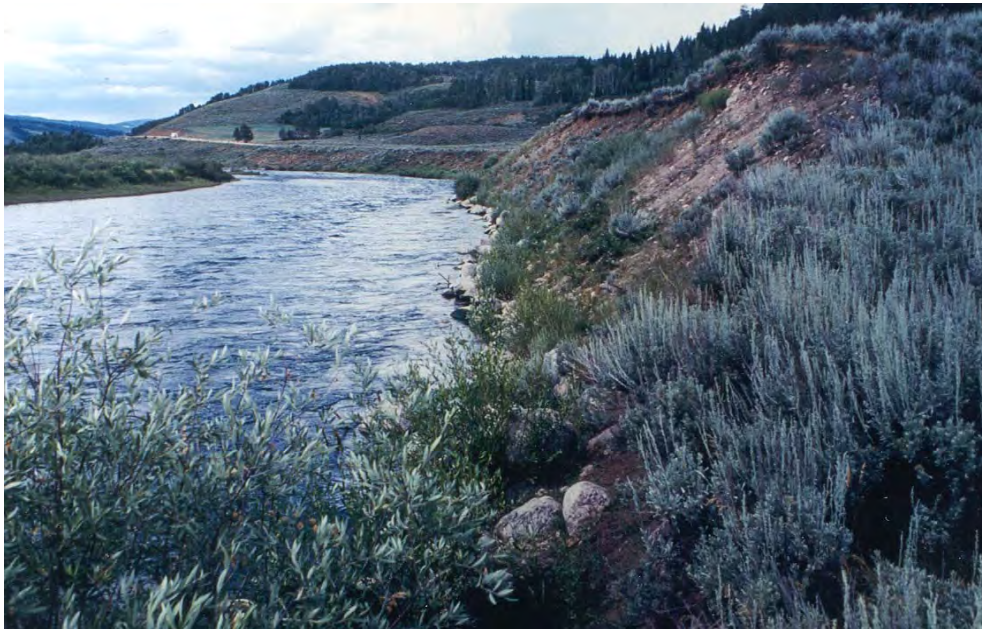
Figure 21-1. Its equilibrium disturbed by channelization downstream on private land, the Green River was actively cutting laterally into this steep bluff located just upstream from the forest boundary. This tree and rock revetment had just been installed when the picture was taken in October, 1988.
