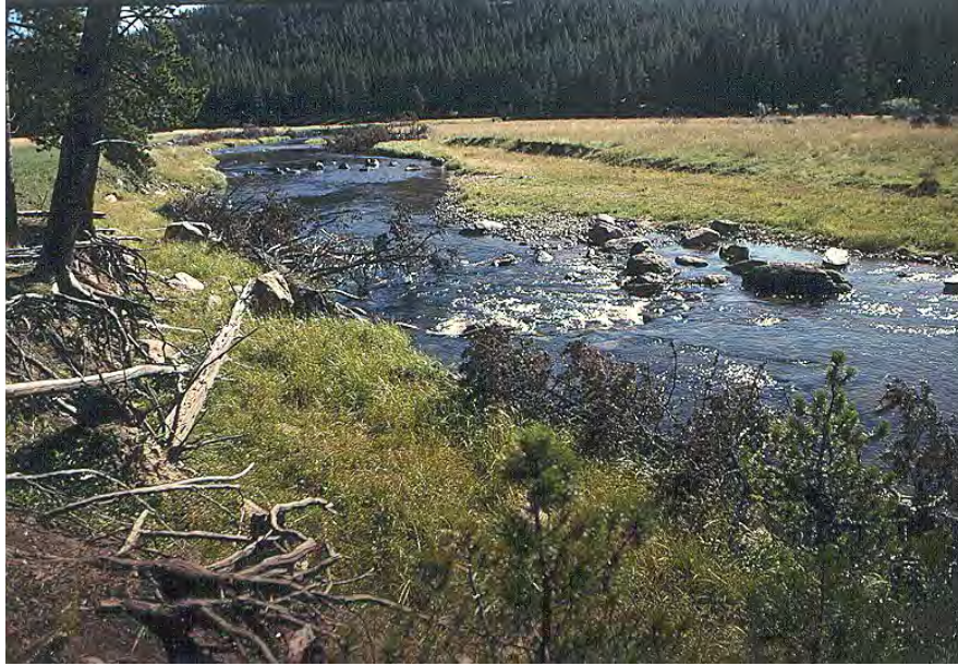
Figure 58-4. Cover trees were anchored next to rock vortex weirs (foreground) to provide shelter for trout using the pools. In this instance, a large trout moved in under the trees before construction was complete, thus demonstrating the need for such habitat. Tree/rock revetments on eroding banks can be seen downstream.
