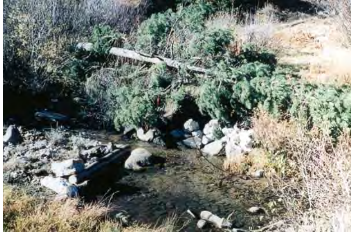
Figure 48-3. Here a combination structure was used in Pass Creek. After the eroding bank was protected with rocks, a conifer was laid over the top to discourage cattle use along that bank. The wing deflector narrows and deepens flow along the face of the rocks, thus increasing cover for trout.
