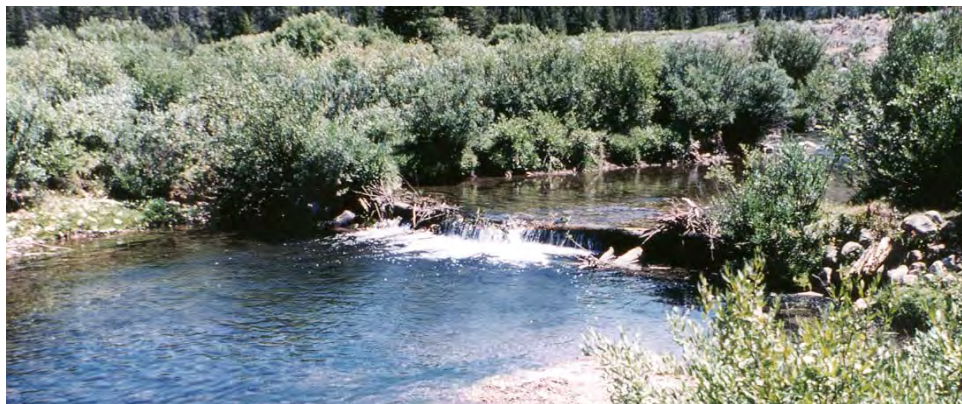
Figure 64-4. A CCC rock crib dam built in 1935 on Tosi Creek was still functional in 1994 and furnishing deep pool habitat for trout.
