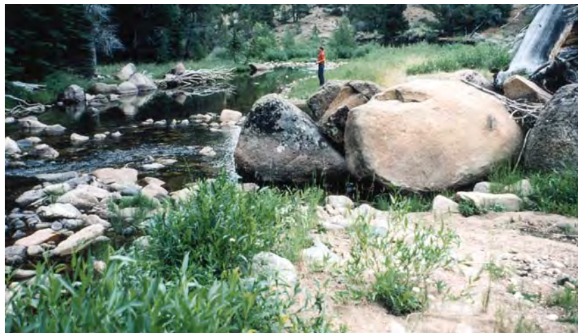
Figure 15-1. A boulder deflector and a tree/rock revetment (far bank) as they appeared soon after construction in 1986.
