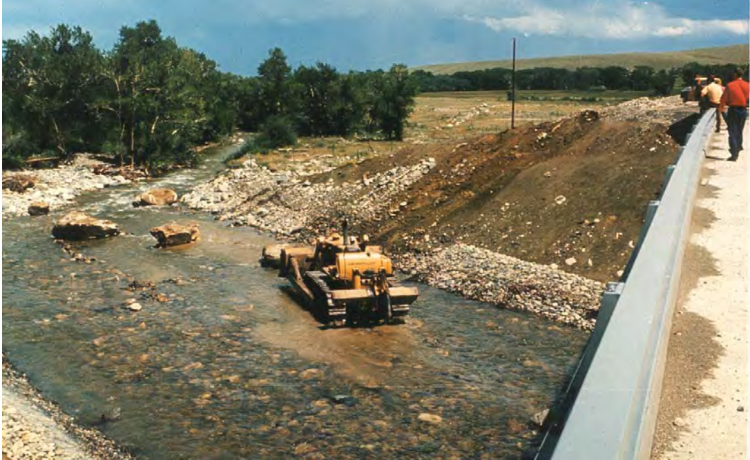
Figure 50-3. As mitigation for channelization done during construction of I-80, 76 large boulders were placed in Rock Creek under the east bridge and upstream from the west bridge crossing. Rock placement extended upstream into the tree-lined section shown in the photo.
