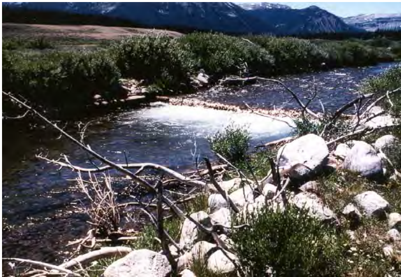
Figure 55-6. A log plunge constructed during Phase I provides both pool habitat and grade control to slow swift flows. Cover trees were installed on both sides of the plunge pool to furnish cover for trout and to make fishing the pool more challenging to anglers.
