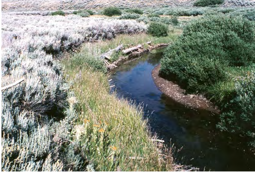
Figure 63-5. A decade after tree revetments were installed, this stream bank is stable. Although some trees near the stream curve are out of the water, the trees in the foreground (note branches protruding from the grass) have formed a grassy berm and offer overhead cover for trout.
