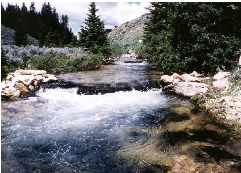
Figure 47-1. Two timber plunges near the confluence with Trail Creek slow swift currents, dissipate energy, and provide deep water to shelter trout.
