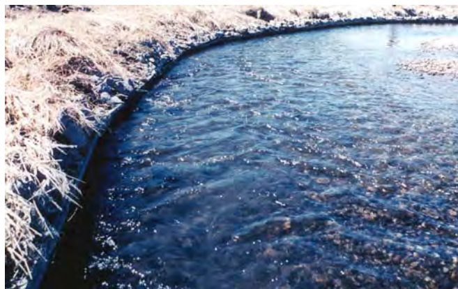
Figure 17-2. Four years posttreatment, a bank protected by skyhook bank panels offers overhead bank cover for trout.
