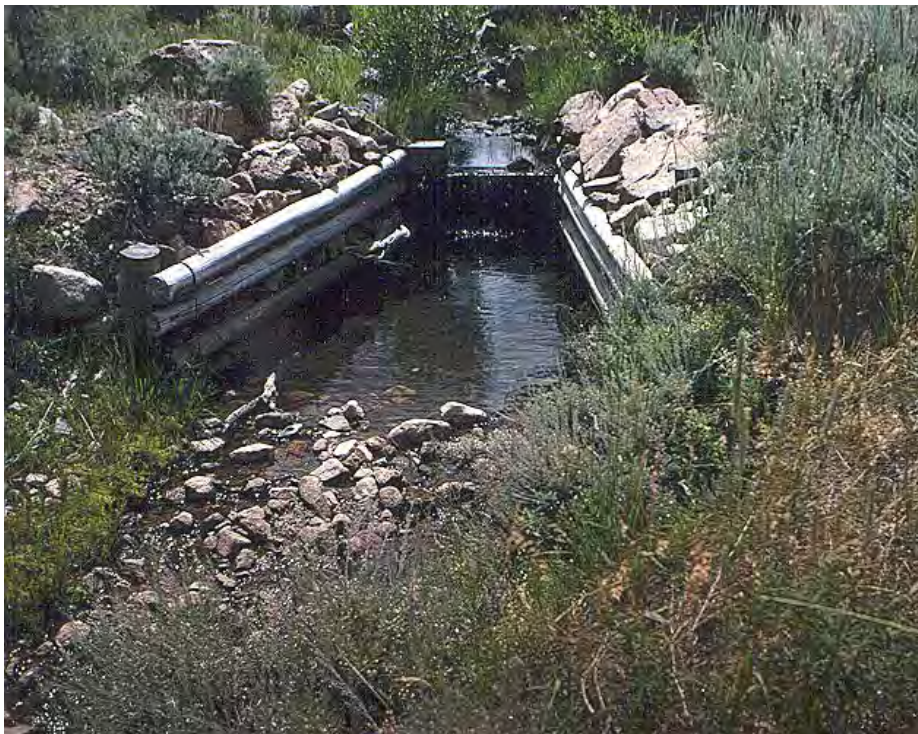
Figure 24-3. A timber plunge at Hall Creek continues to furnish deep pool shelter for juvenile trout 11 years after installation.
