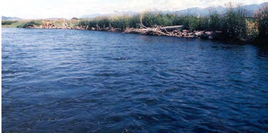
Figure 54-4. Several years after a tree revetment was installed, this formerly eroding bank is very stable. Note the dense growth of willows that has developed along the bank behind the trees.
