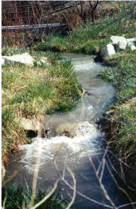
Figure 68-1. A timber plunge (top of photo) and a rock plunge (foreground) slow flows in Wolf Creek and provide pool habitat for fish.
