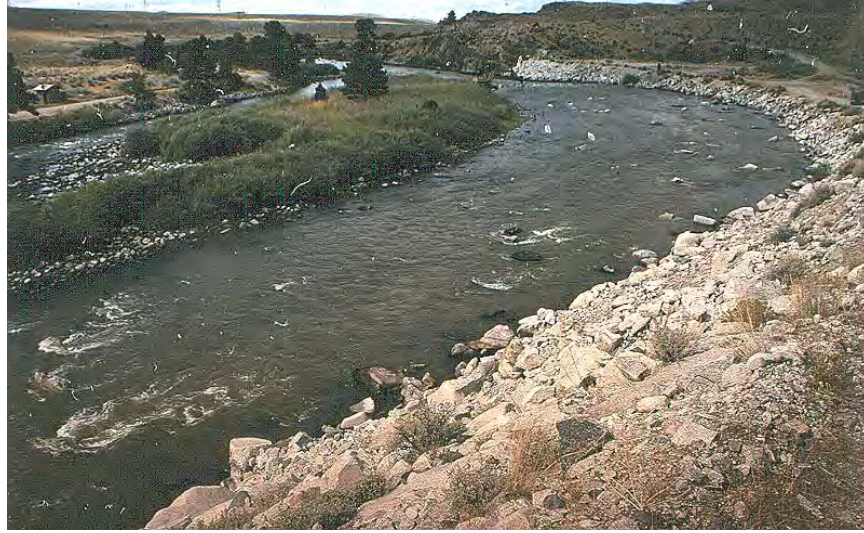
Figure 45-1. Large boulders were added to a swift section of the river to supplement fish cover provided by several existing boulders.
