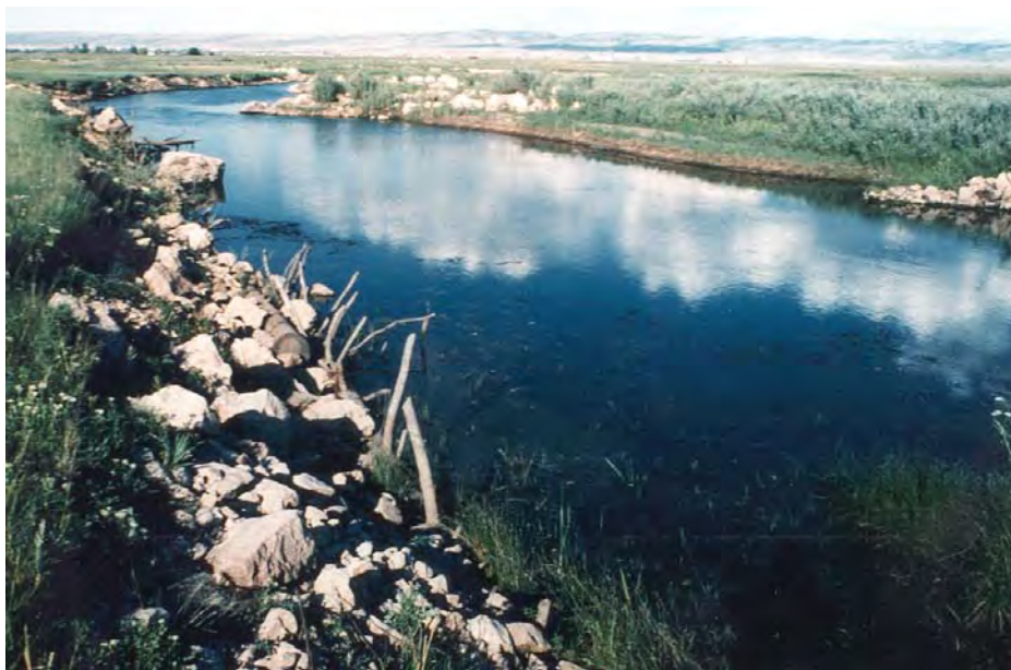
Figure 33-3. Eight years after this tree/rock revetment was built, stream banks are stable and there is cover for trout along the deep interface of trees and water. Willows and other riparian vegetation have established on the point bars and along the banks.
