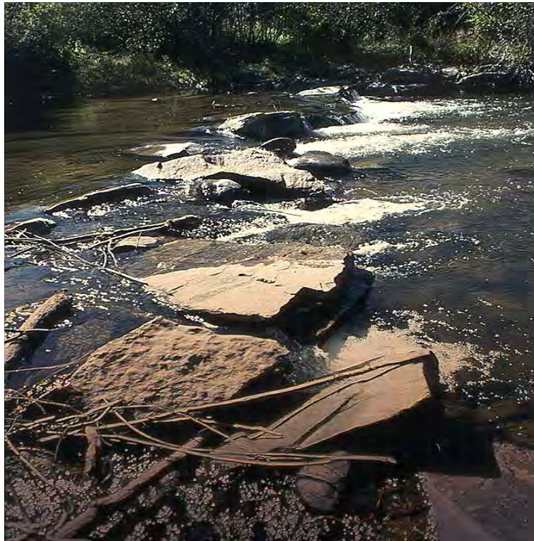
Figure 5-2. Close-up view of a boulder weir at Big Creek, which created pocket pools, a dam pool, and a plunge pool. These weirs also acted as grade controls and helped increase subirrigation of the riparian zone.
