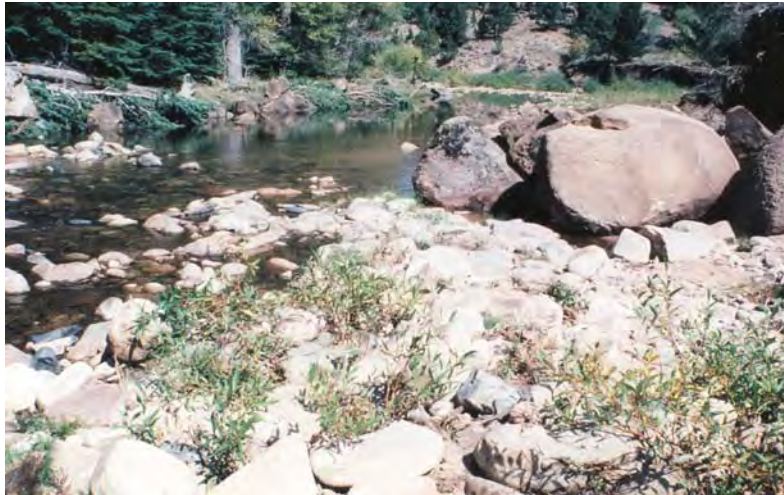
Figure 15-1. A boulder deflector and a tree/rock revetment (far bank) as they appeared soon after construction in 1986.
