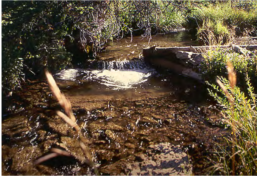
Figure 18-1. Rocks and logs were added to this wing deflector to create a plunge, which is controlling grade and providing plunge pool shelter for trout.
