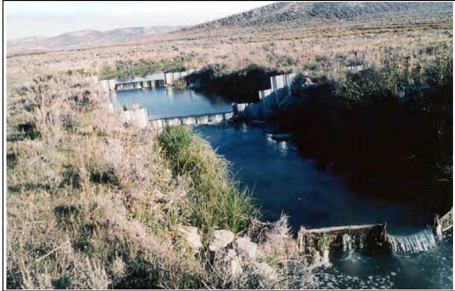
Figure 39-1. A series of three plunges made from C-LOC brand PVC plastic panels provides deep pools for fish, grade controls, and elevated water level to better subirrigate the stream banks on lower Muddy Creek.
