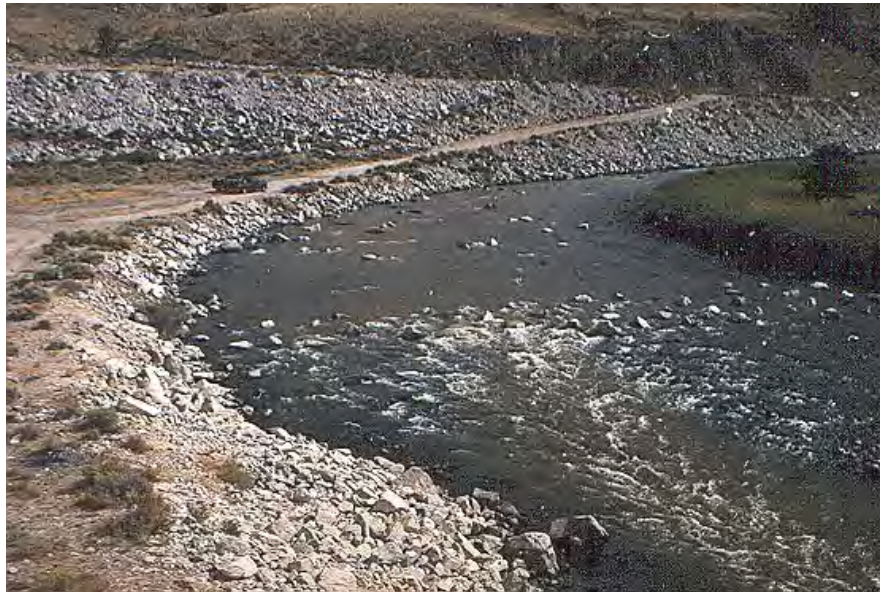
Figure 45-2. A loose rock sill was constructed to act as a grade control, raise water levels in the upstream river, and provide additional shelter for fish.
