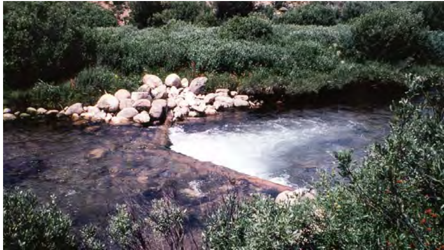
Figure 64-6. An upstream "V" plunge built by WGF was in good condition 12 years after construction. It was furnishing both shelter to trout and a grade control to slow swift stream flows in this section.
