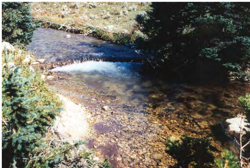
Figure 47-2. A log vortex weir (upstream “V” plunge) acts as a grade control to slow stream flow and furnishes valuable pool shelter for trout.
