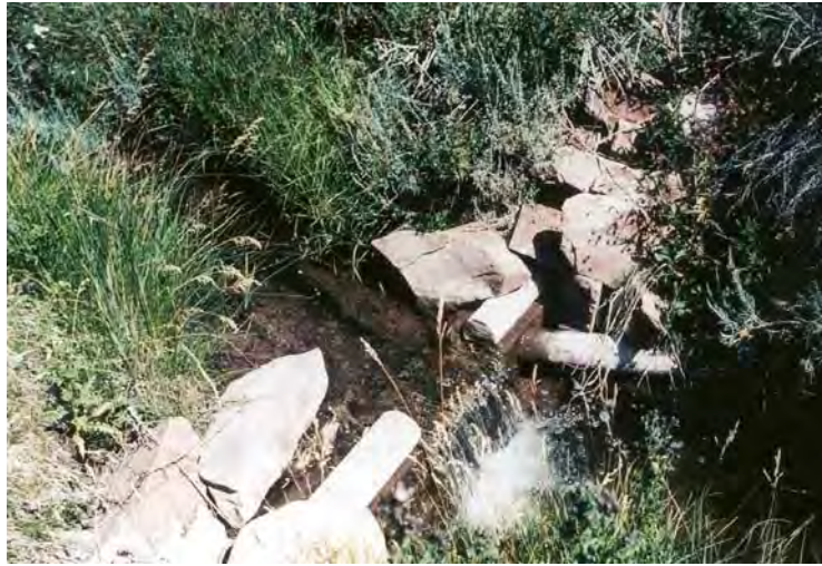
Figure 49-1. Timber plunges installed in Pinegrove Creek have provided shelter for trout, grade control for the stream, and subirrigation for the riparian vegetation.
