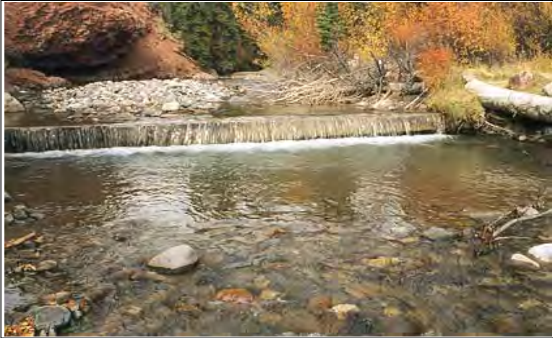
Figure 1-2. A log plunge located near the mouth of Bear Creek Canyon provides deep pool shelter for trout and helps dissipate energy during high flow events.
