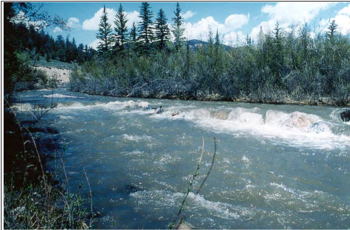
Figure 1-1. A boulder S-dam installed in Bear Creek slows swift spring flows and provides shelter for trout.
