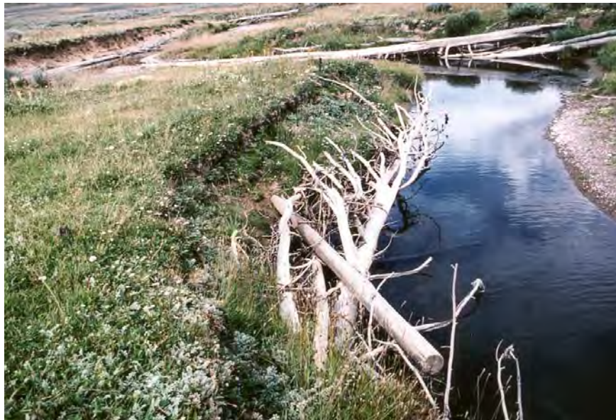
Figure 63-6. This photo shows the contrast in effectiveness of the tree revetments. In the foreground, the bank is stable with woody debris shelter offered trout by the trees. However, at the top of picture, left, the bank there is still unstable and the trees were not effective at preventing bank erosion.
