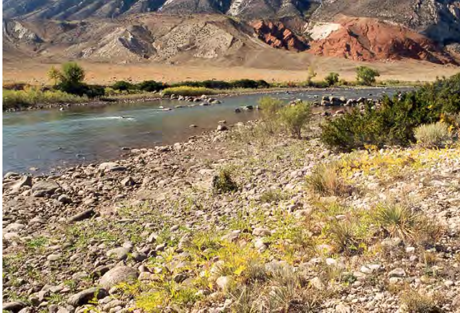
Figure 12-1. Two lines of boulders created a rock funnel to provide pool shelter and habitat diversity for fish in the Clarks Fork River. Instream fish rocks downstream from the slot of the funnel provide additional shelter.
