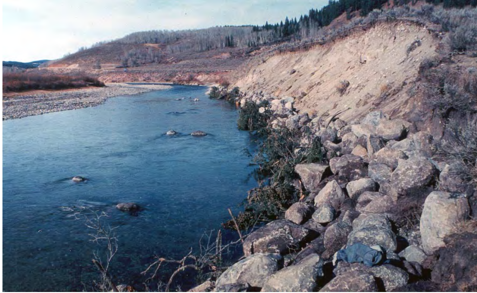
Figure 21-1. Its equilibrium disturbed by channelization downstream on private land, the Green River was actively cutting laterally into this steep bluff located just upstream from the forest boundary. This tree and rock revetment had just been installed when the picture was taken in October, 1988.
