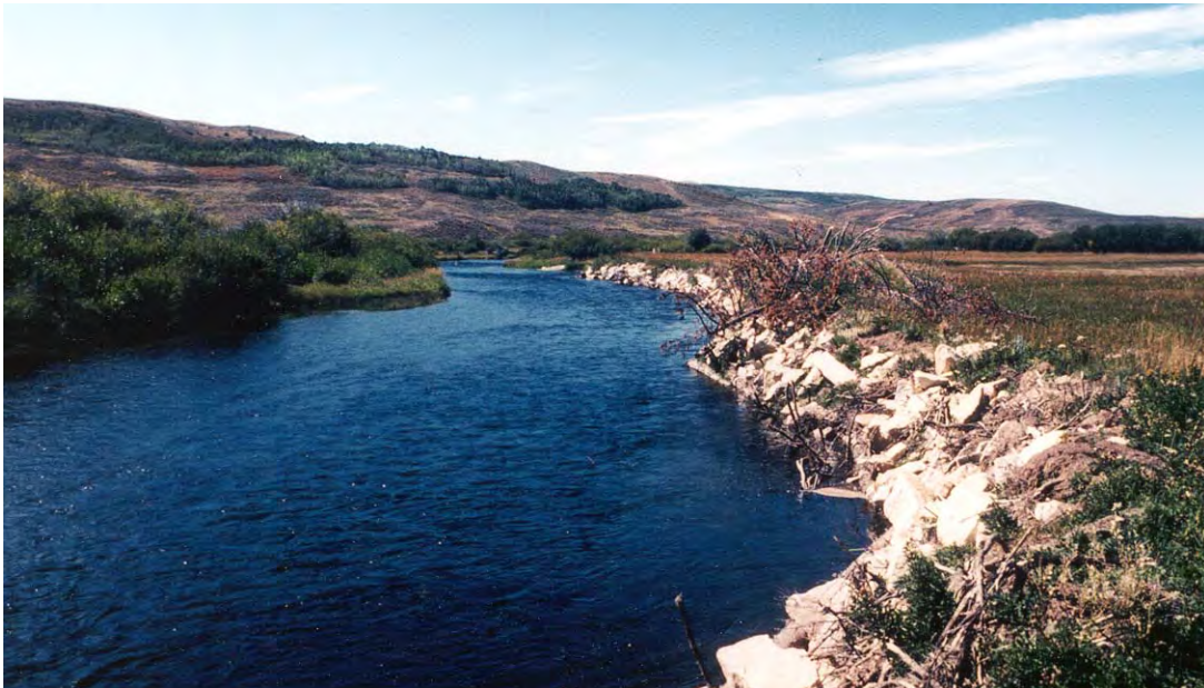
Figure 25-1. Many unstable stream banks on the Peternel PFA were stabilized with tree and rock revetments, which also provide shelter for trout along stream edges.
