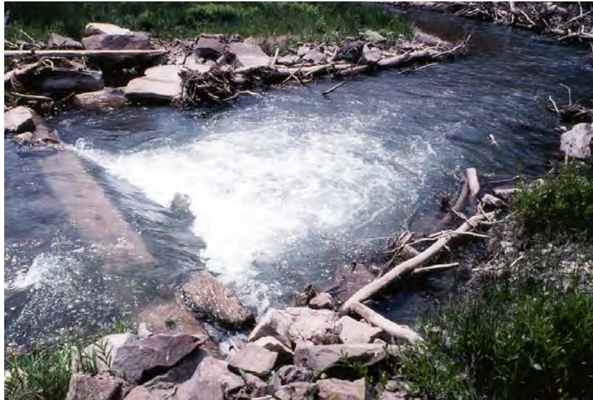
Figure 53-1. A log plunge installed in Salt Creek provided both grade control and shelter for trout. But by 1997, the plunge pool had migrated downstream to form a deep corner pool along the face of the tree/rock revetment (top of picture, right).
