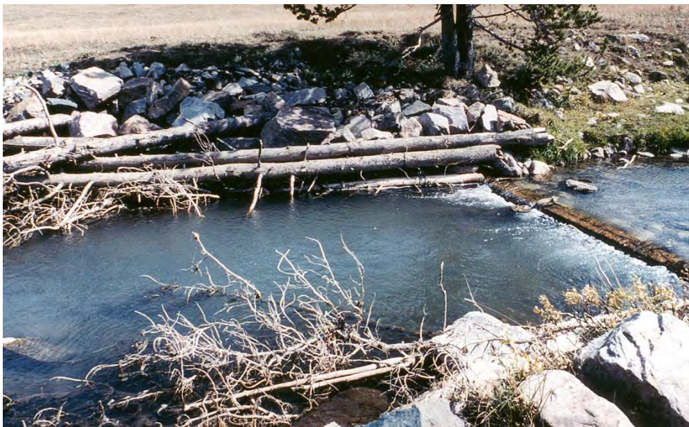
Figure 35-2. This is the same site shown in Figure 35-1 after a timber plunge and a tree/rock revetment were added. Provision of a deep plunge pool adds a key element for overwinter survival of trout.
