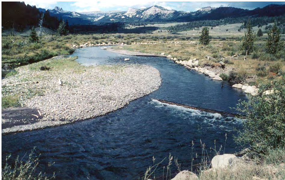
Figure 28-3. Four years posttreatment, instream digger log barbs and tree/rock revetments have reduced erosion of banks and stabilized the channel in the meadow at Horse Creek.
