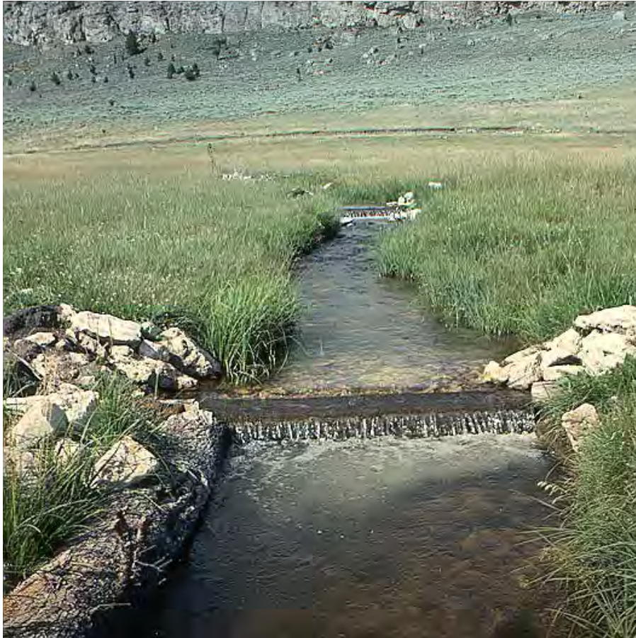
Figure 3-2. To provide deep pool cover for trout, as well as to help subirrigate the riparian vegetation, 58 pool digger structures were installed at Beartrap Meadows.
