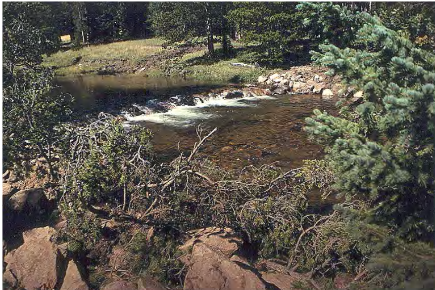
Figure 58-3. Diagonal rock weirs were also constructed to create deep pools and control stream grade.
