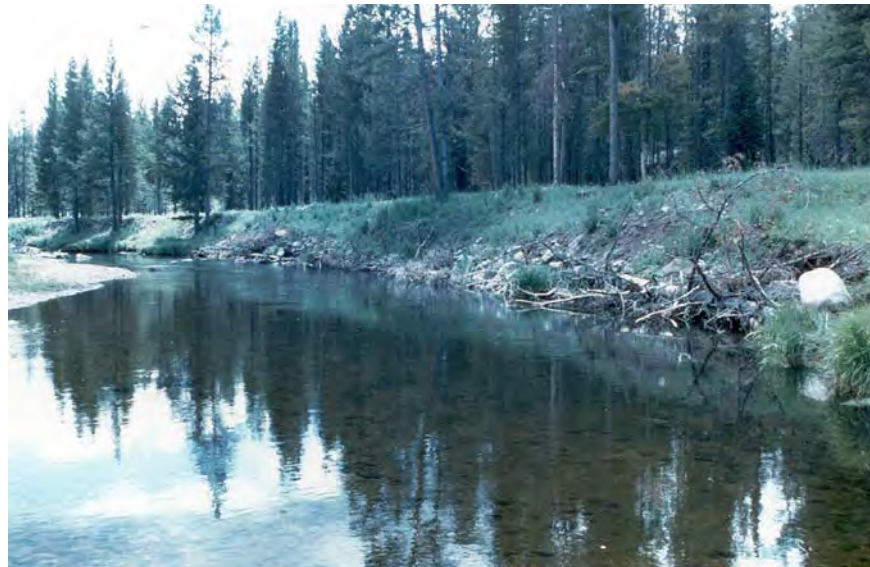
Figure 56-4. Pretreatment, this bank was being severely eroded by the river, but ten years after a tree/rock revetment was installed, the bank is completely healed. When this section is electrofished, many trout are found living in the deep pools and woody debris along the bank.
