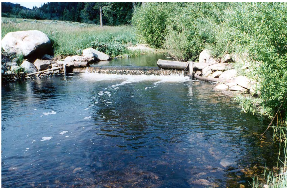
Figure 30-1. A log plunge still provides deep pool shelter for trout in LaBonte Creek 11 years after it was built. RPD was over 4 ft in this pool.
