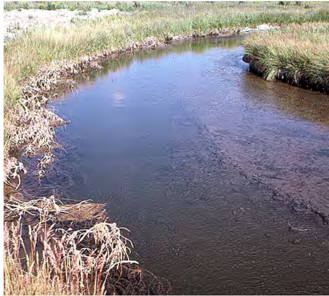
Figure 17-1. A bank protected with a tree revetment as it appeared six years posttreatment. A deep slot was excavated in the channel along the tree edge when the trees were installed.
