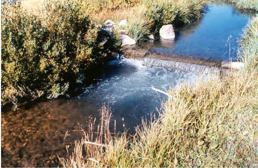
Figure 10-3. Timber plunges installed in Bull Creek provided both plunge pools and dam pools to shelter trout.
