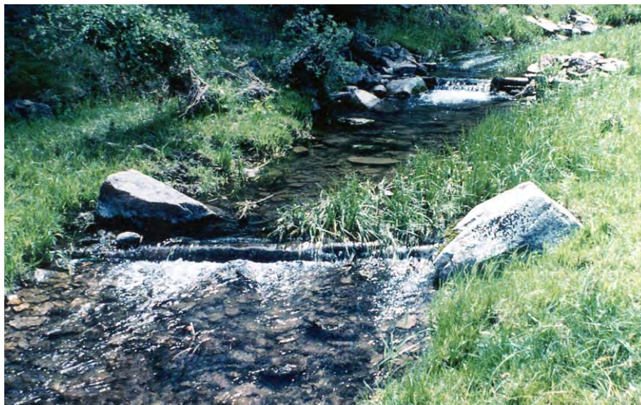
Figure 4-2. This timber plunge at Beaver Creek had a log grade control to maintain pool depth.
