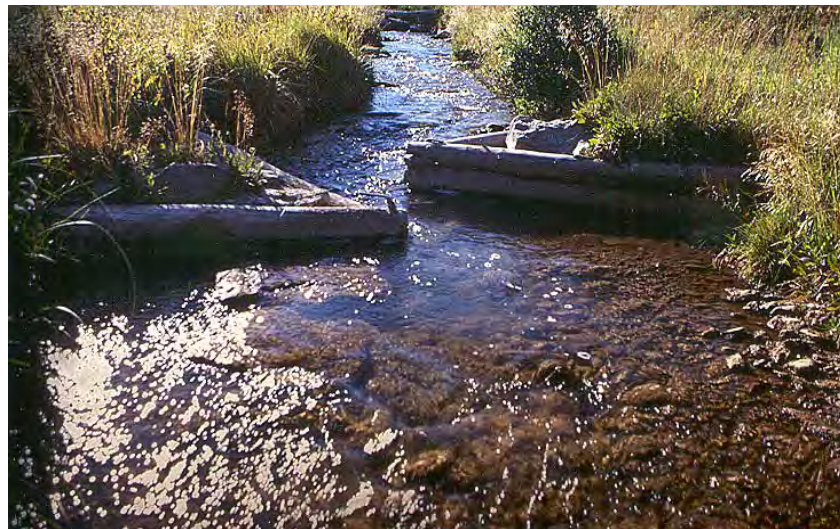
Figure 18-4. Offset double deflectors increased habitat diversity in Fool Creek and provided some overhead cover near deflector tips, but no deep pool shelter formed.
