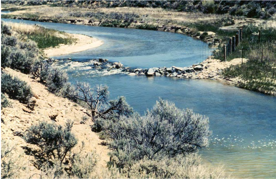
Figure 6-2. A boulder weir on the Big Sandy River turns the flow into a rocky bluff to create better shelter for trout. A livestock exclosure is at top right.
