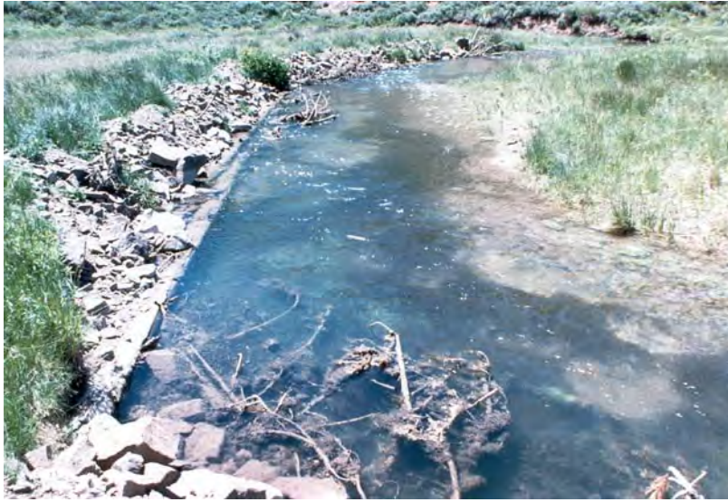
Figure 53-5. Tree and rock revetments stabilized eroding banks, provided deep pool habitat, and many of the logs furnished overhanging bank shelter for trout.
