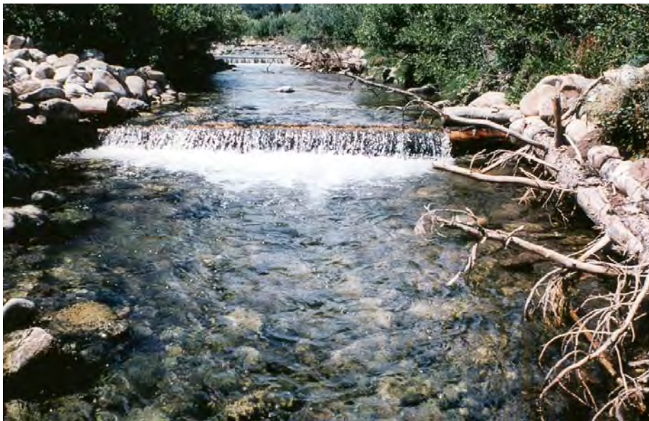
Figure 51-2. Log plunges were built in Rock Creek to provide grade control and furnish pool shelter to trout. Cover trees placed along the sides of plunge pools added both cover and structural stability.
