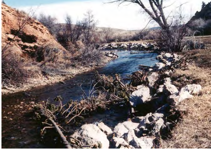
Figure 36-2. This tree/rock revetment was built during Phase II to stabilize an eroding stream bank, slow swift currents on an extended riffle, and provide cover for BNT.
