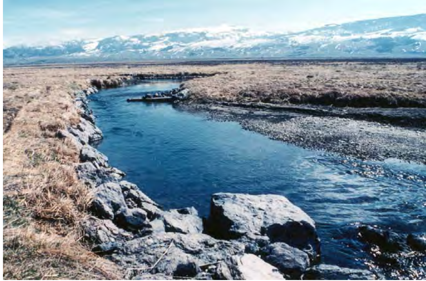
Figure 17-3. Rock riprap was used to stabilize only a few banks at Flat Creek. Five years posttreatment, the rocks retain their original configuration and the wing deflector has caused the low flow channel to narrow as sediment has deposited in a bar downstream from the deflector.
