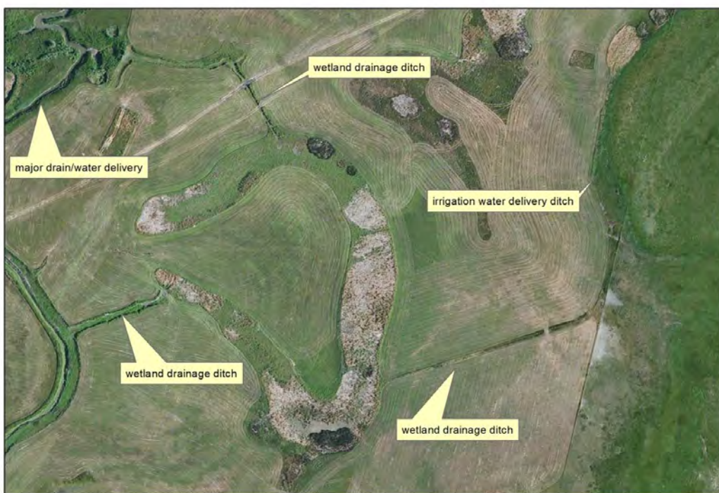
Fig 15. Aerial photo of drainage and water delivery ditches in an irrigated field, Bear River complex.
