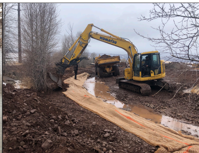
Figure 69. Swift Creek stream restoration.
