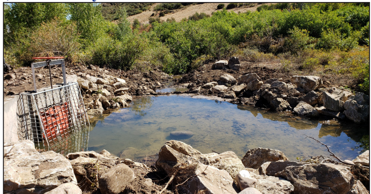
Figure 14. Mule Creek headgate.
