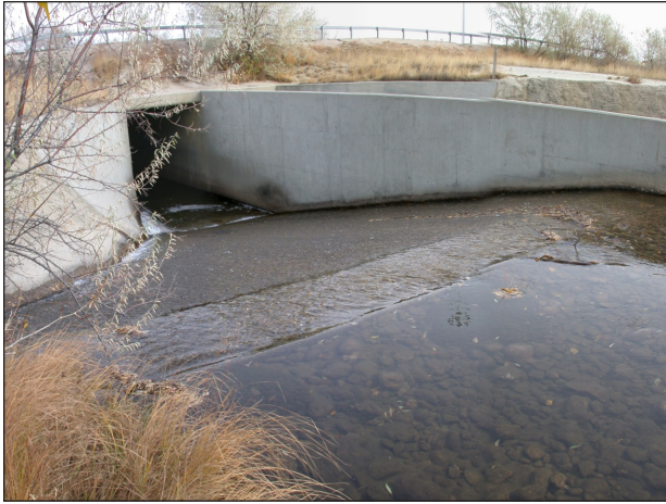
Figure 151. Grade control structure and fish barrier located on Clear Creek upstream of Interstate-25.
