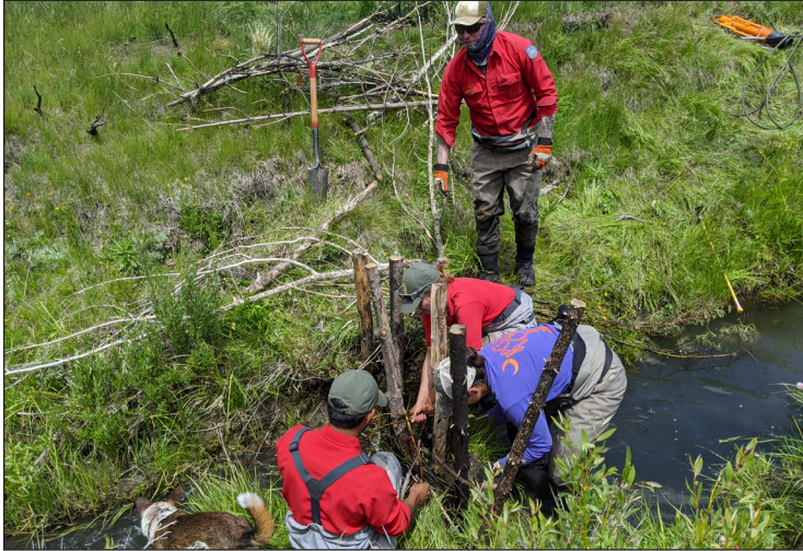
Figure 65. WGFD and Bridger Teton USFS crew installs a beaver dam analog on Little Horse Creek.
