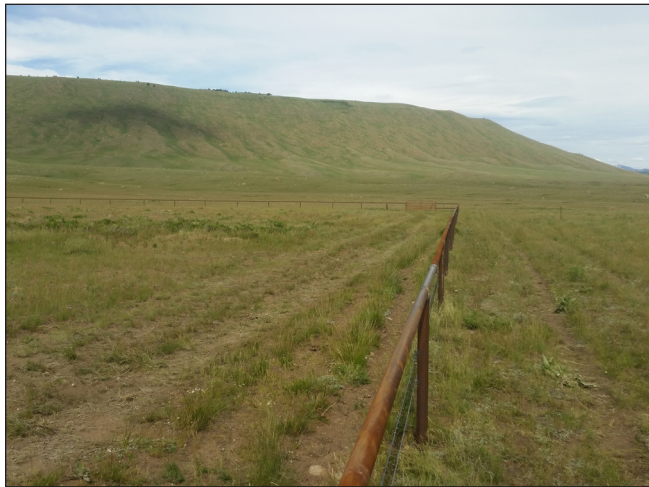
Figure 126. New drill stem wildlife friendly fence.
