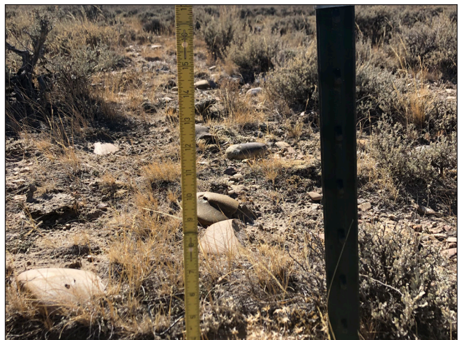
Figure 124. Addition of a smooth bottom wire and raising height to 18 inches off the ground.
