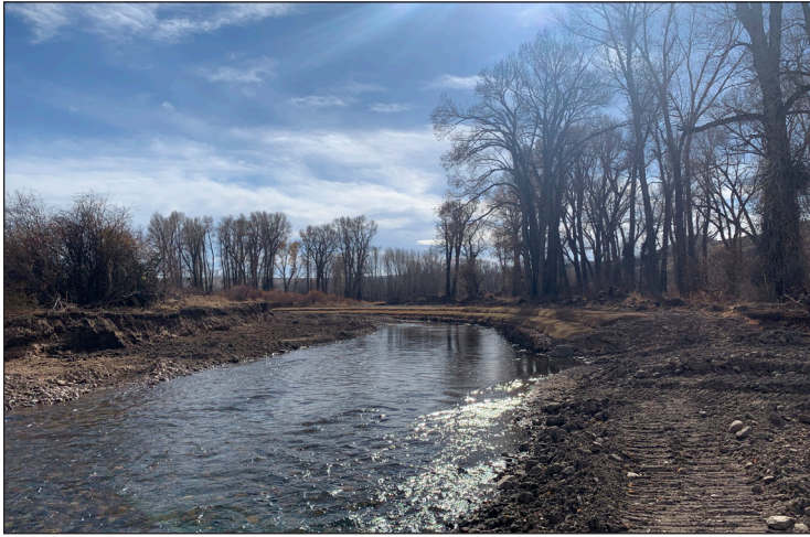
Figure 101. Completed toewood and bankfull bench along new channel alignment.
