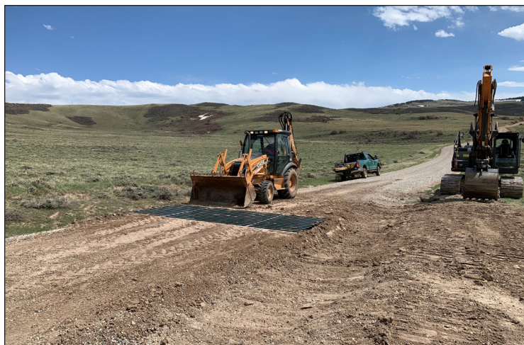
Figure 115. Statewide crew installing new cattle-guard where an electric fence will go.
