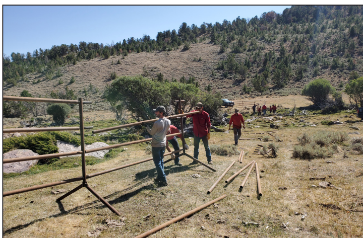
Figure 26. Assembly of steel jack fence on Sanchez Creek.
