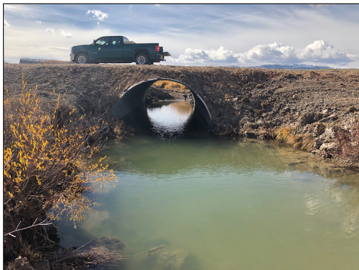
Figure 11. Little Cottonwood Creek culvert after construction.
