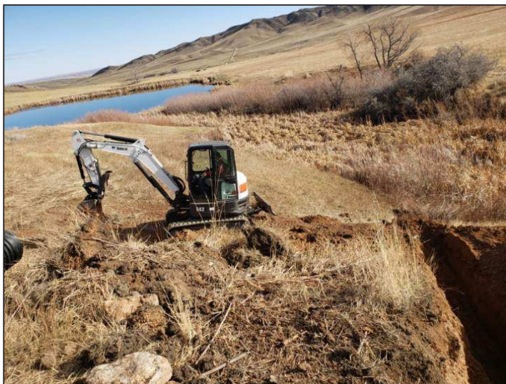
Figure 12. AgriDrain installation on Sayles Reservoir No. 2.
