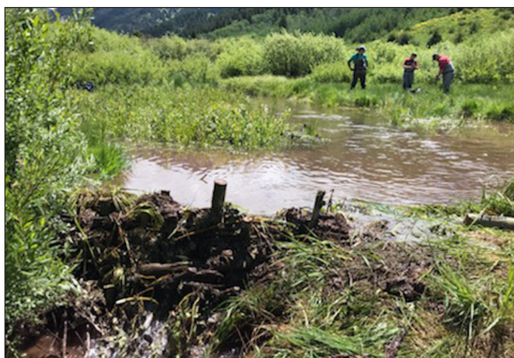
Figure 67. A completed and impounded BDA on Muddy Creek.
