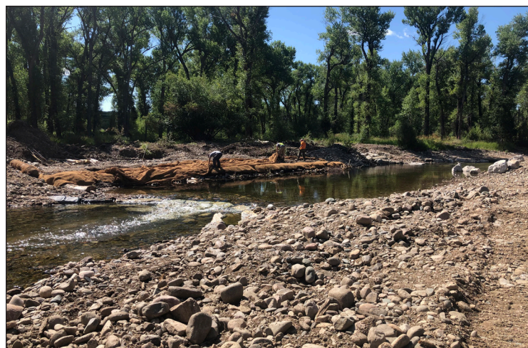
Figure 109. Installing soil lifts along toewood treatments.
