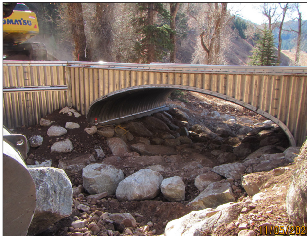
Figure 4. Looking downstream at bottomless arch crossing and rock ramp.
