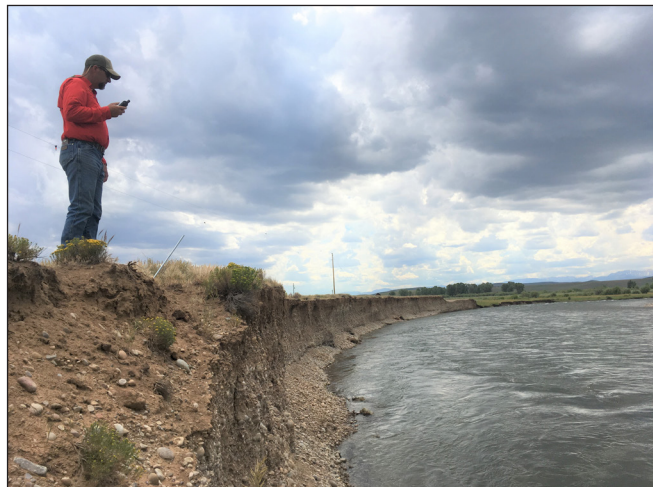
Figure 122. Vertical eroding stream bank at the Daniel/40-Rod Access.
