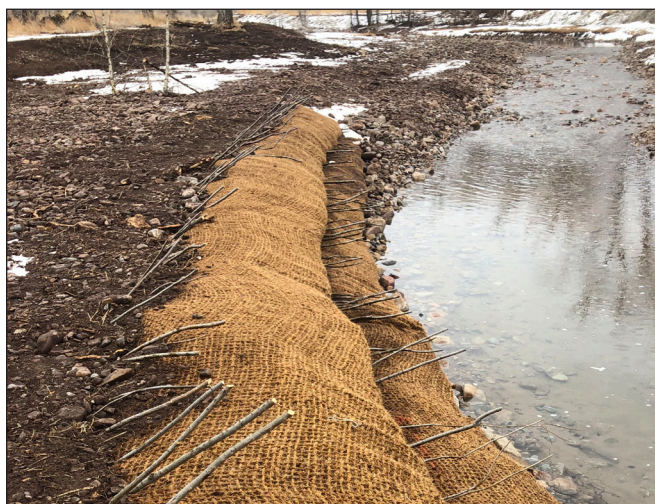
Figure 68. Swift Creek soil lifts.
