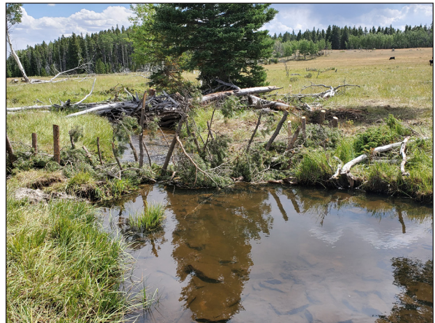
Figure 156. Installing a BDA structure.
