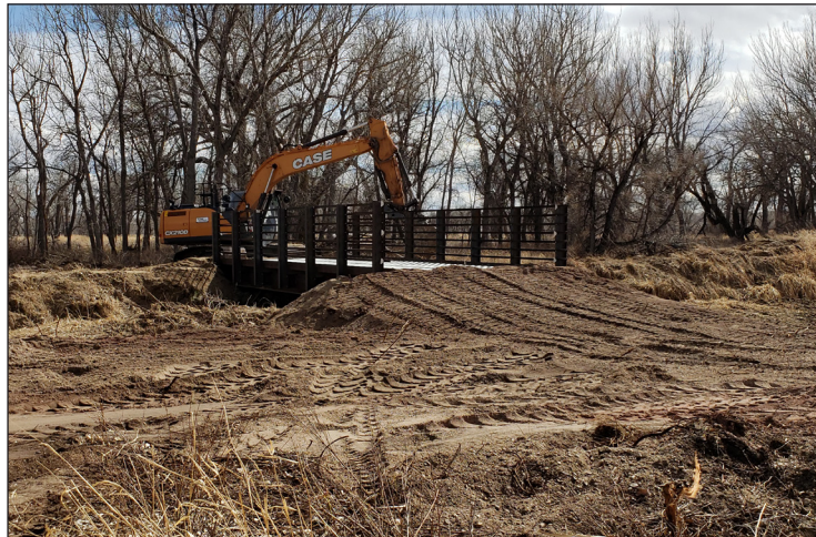
Figure 108. Rawhide WHMA Bridge installation.
