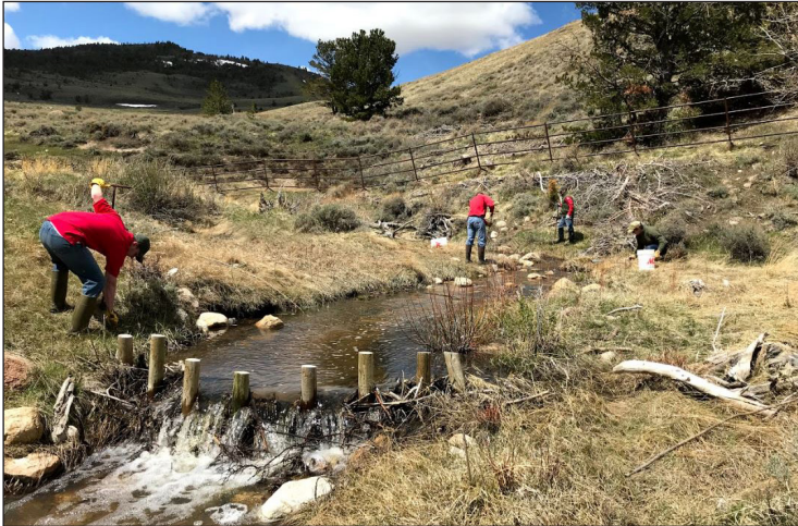
Figure 87. Willow plantings on West Cottonwood Creek in the reach where BDAs were installed.
