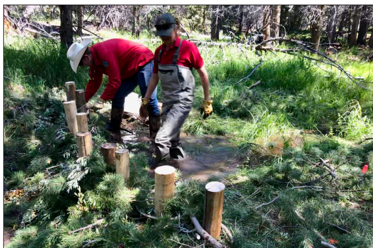
Figure 76. Installation of BDA's on Mill Creek in the Shoshone National Forest.
