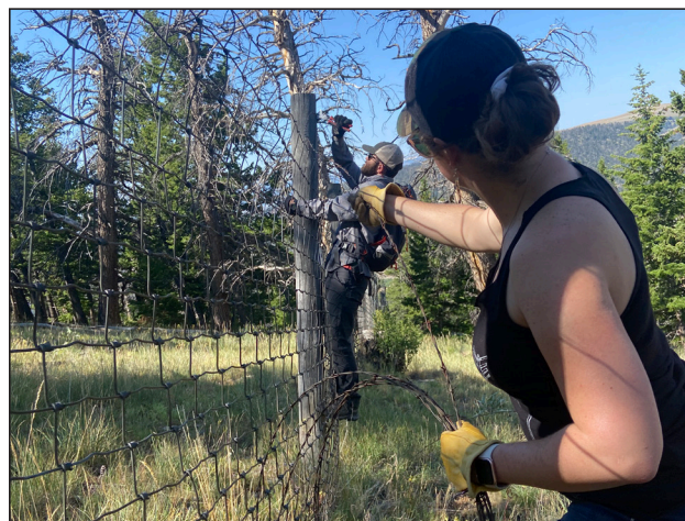
Figure 75. Volunteer crew working to remove fencing from Elk Ridge.
