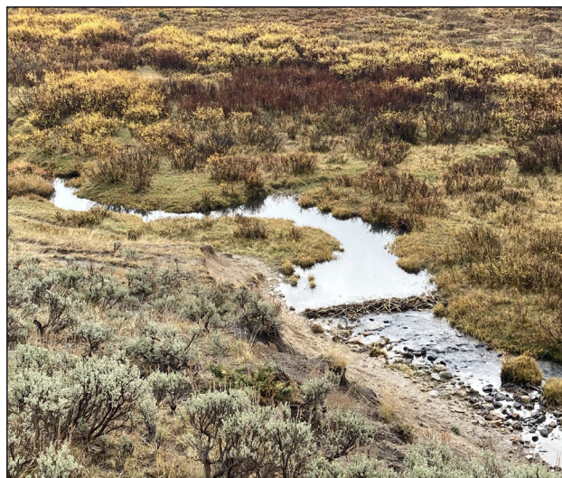
Figure 20. Newly constructed dam on Buckskin Ed Creek. Cody Regional Office property in 2023. These efforts have been made possible by a generous, private donation.
