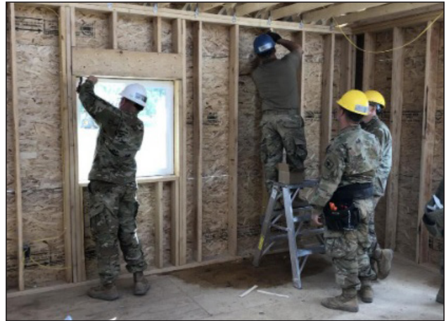
Figure 117. Wyoming Air National Guard framing a bunkhouse.
