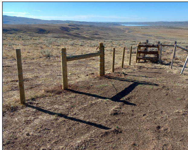
Figure 38. Fences converted to wildlife friendly fencing standards.
