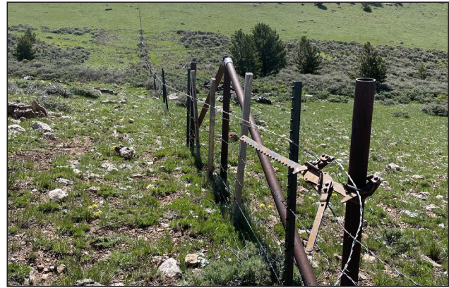
Figure 150. North fireproof fence.
