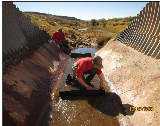
Figure 49. Installing rubber baffles.
