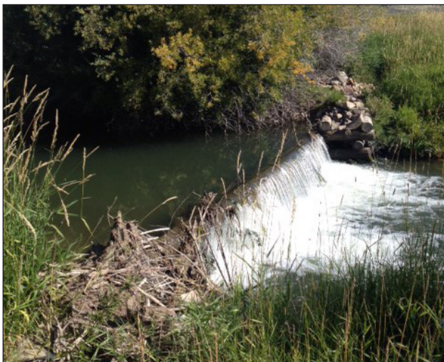
Figure 43. Diversion before improvements.
