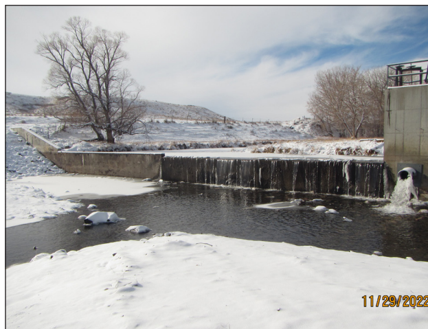
Figure 103. Completed Burger Diversion.
