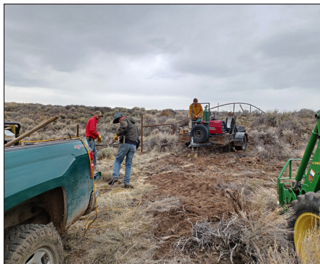
Figure 131. Installing wildlife friendly fencing.
