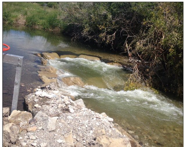
Figure 44. Diversion after improvements.
