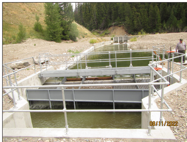
Figure 69. Looking upstream at fish screen and sediment settling basin.
