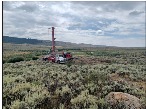
Figure 133. Well drilling at Soda Lake Wetlands.
