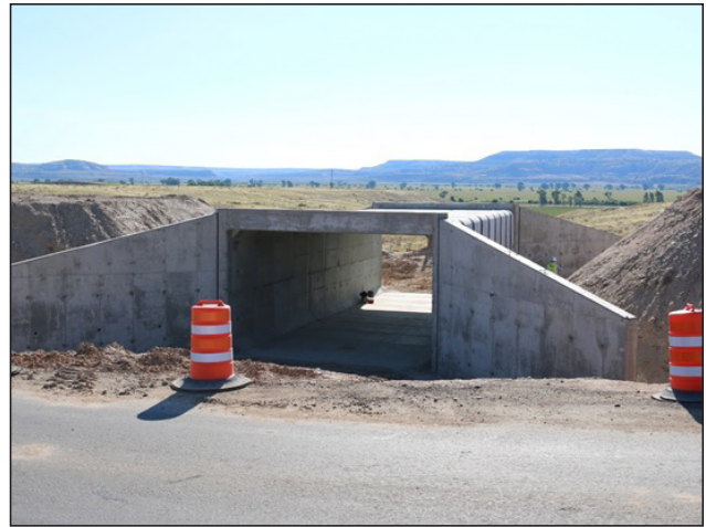
Figure 119. Box culvert underpass constructed on the Dry Piney Wildlife Crossing project.
