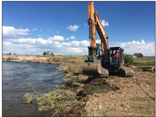
Figure 118. Installing toe wood.
