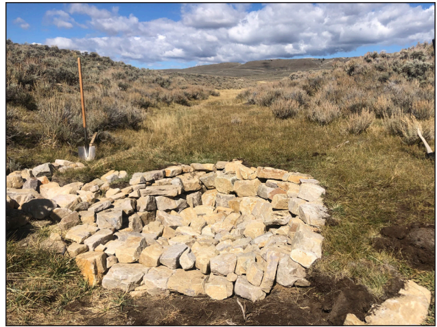
Figure 126. Completed Zuni Bowl structure within Monument Draw.
