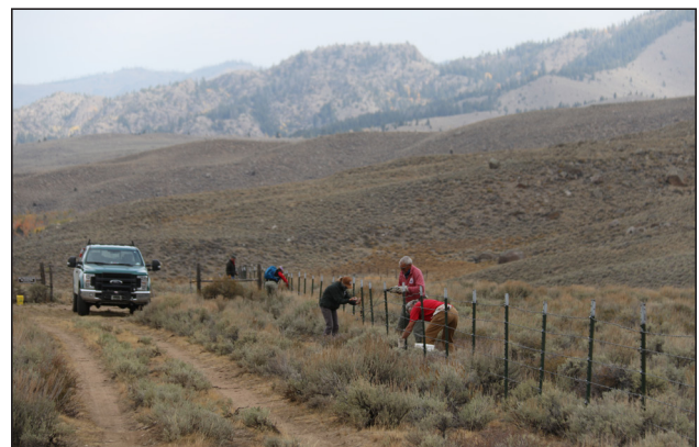
Figure 139. Partners and volunteers work to modify an existing fence.
