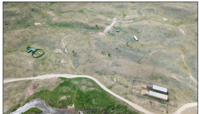
Figure 120. Overview of solar well and water tanks at Fall Creek WHMA.
