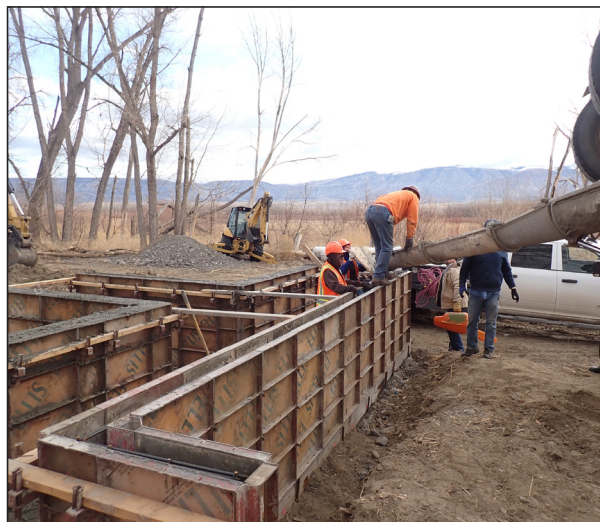
Figure 30. Installing a concrete diversion box.
