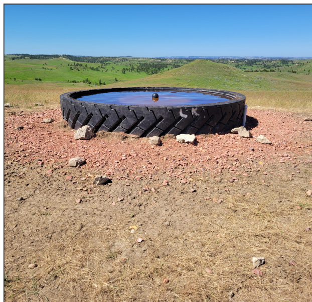
Figure 158. Water tank installed.
