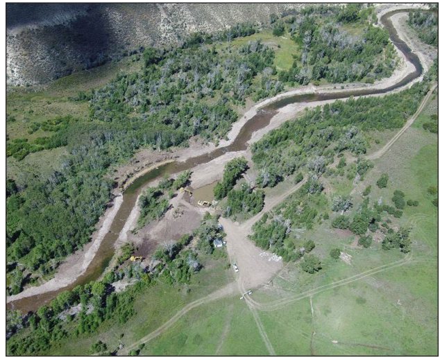
Figure 42. Aerial view of Evanston Dam rehabilitation reach.
