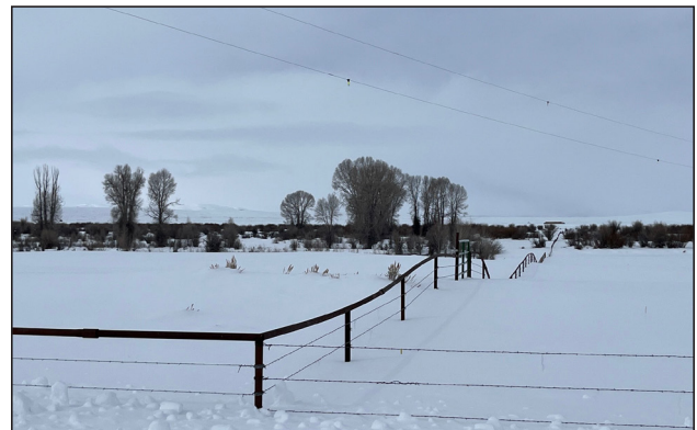
Figure 122. 40-Rod pipe boundary fence.
