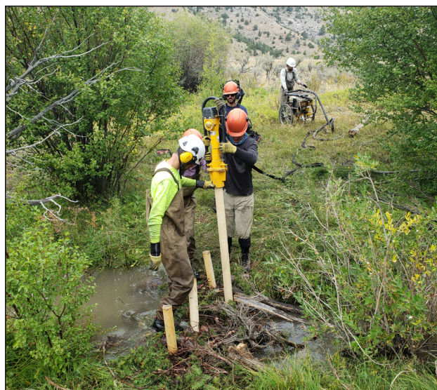
Figure 24. Installation of a BDA on Enos Creek.
