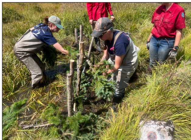
Figure 92. Building a BDA on Fall Creek.
