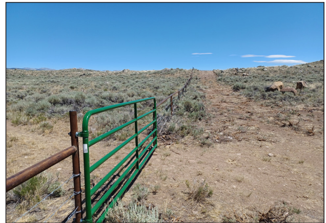
Figure 125. Completed wildlife friendly pipe fence on Luke Lynch WHMA boundary.
