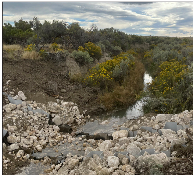
Figure 5. Bolton Creek Sheet Piling structure.
