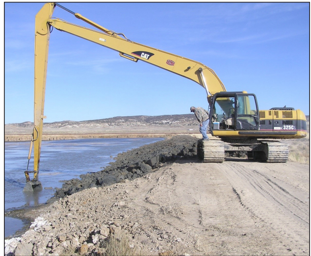
Figure 58. Duck Pond No. 5 rehabilitation.
