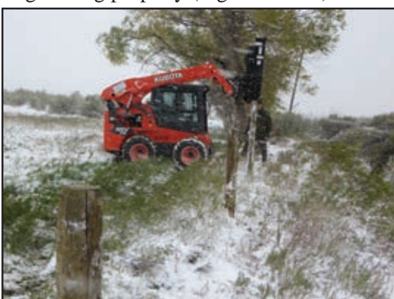
Figure 41. New fence posts being installed.
