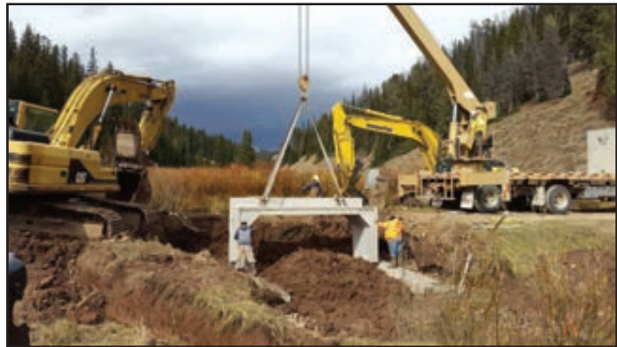
Figure 6. New concrete bottomless arch culvert, October 2016.
