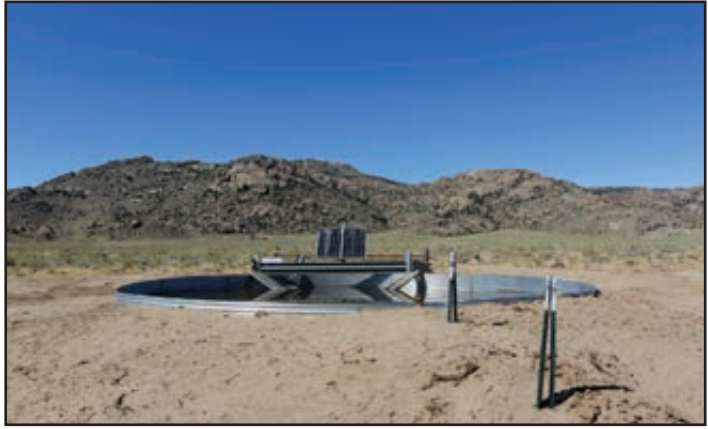
Figure 96. Conversion of a dilapidated windmill to a solar pump with a new tank near Sweetwater Rocks to benefit mule deer, sage grouse, and pronghorn.
