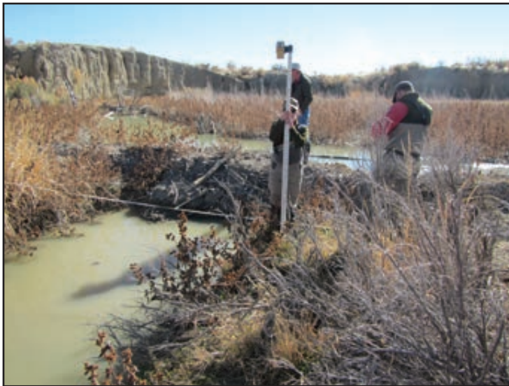
Figure 18. Surveying a Bolton Creek cross section downstream of a BDA.
