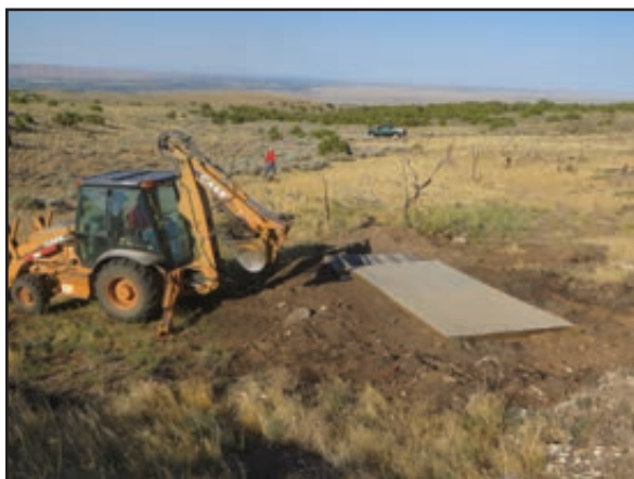
Figure 39. Little Mountain guzzler before back filling.
