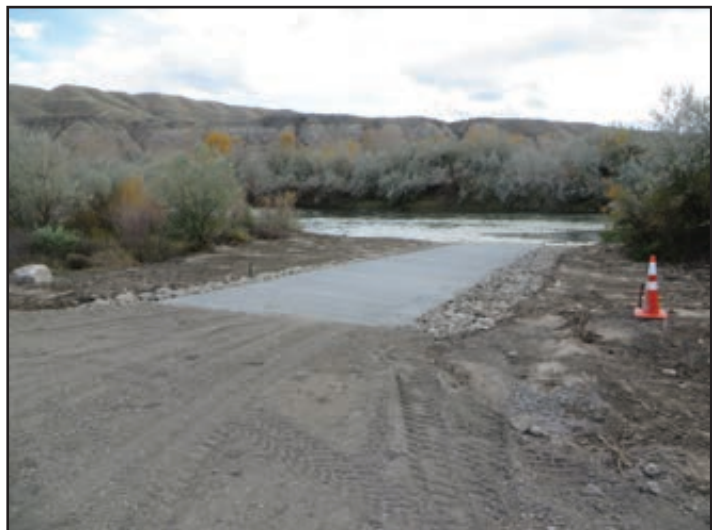
Figure 50. New concrete boat ramp at Corbett Bridge on Shoshone River.
