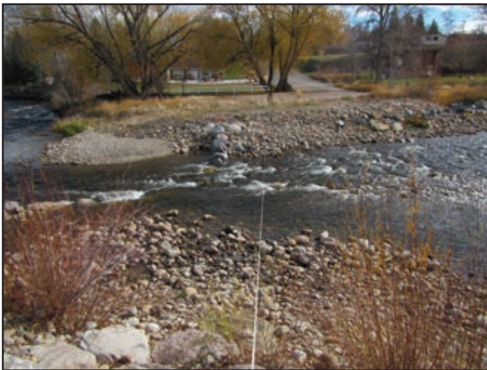
Figure 107. Surveying a cross section upstream from a structure that will receive maintenance in 2017.
