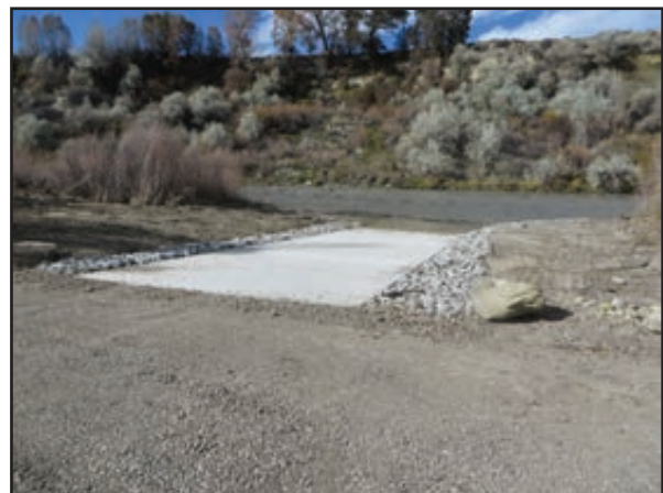
Figure 53. New concrete ramp at Willwood Dam on the Shoshone River.
