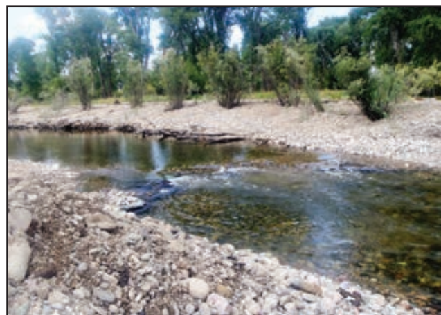
Figure 123. Upstream end of reconstructed rock constructed riffle with newly transplanted willows on riverbank at the Encampment River - Boykin maintenance.
