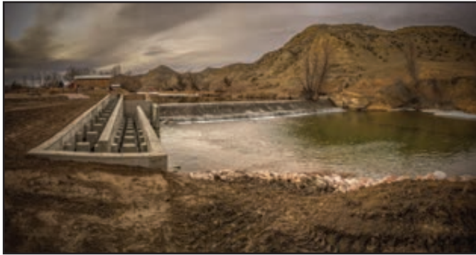
Figure 177. Dual vertical slot fish ladder (left) located between the Pratt and Ferris #1 dam and diversion ditch. Photo on right depicts a close-up view of the operating ladder.
