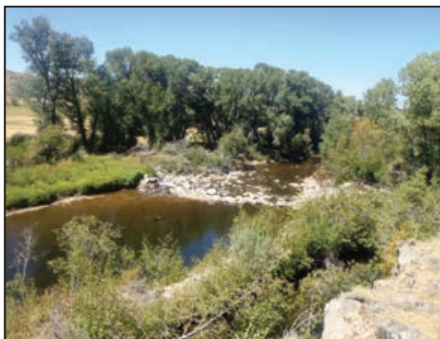
Figure 120. Wagoner Diversion on the Encampment River before replacement.
