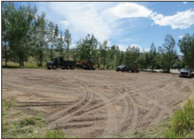
Figure 65. New parking lot looking from the Southeast corner.
