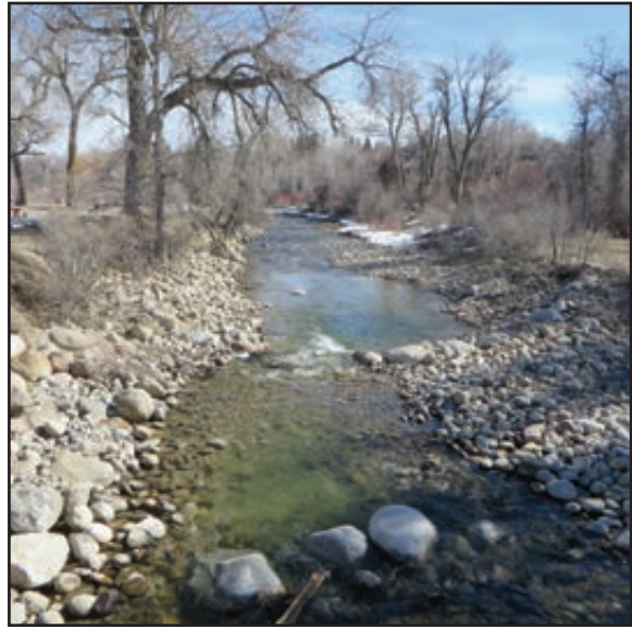
Figure 106. An excavated low flow channel and boulder features enhance trout habitat on the Middle Popo Agie River.
