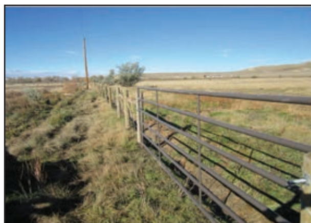
Figure 42. Completed boundary fence on Yellowtail WHMA.
