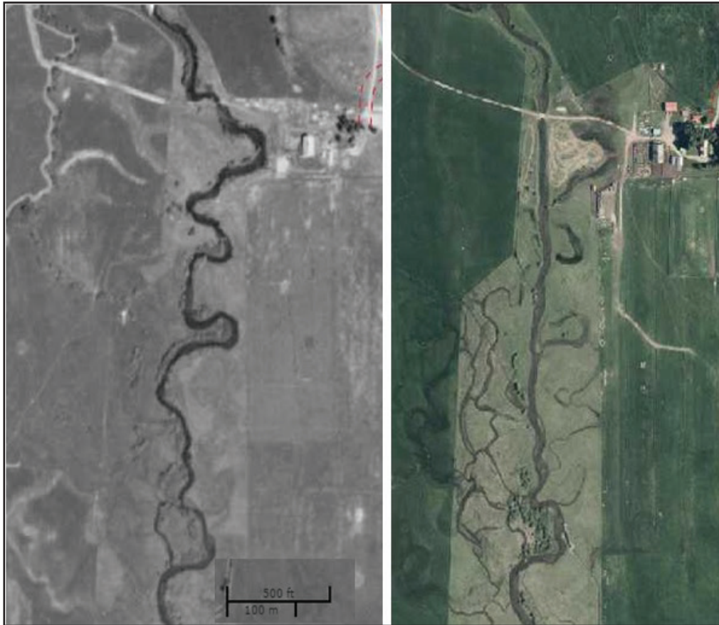
Figure 89. Flat Creek from 1945 (left) and 2015 (right) show channel straightening and willow removal.
