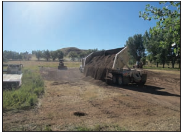
Figure 66. 20 yard side dump delivering road base
