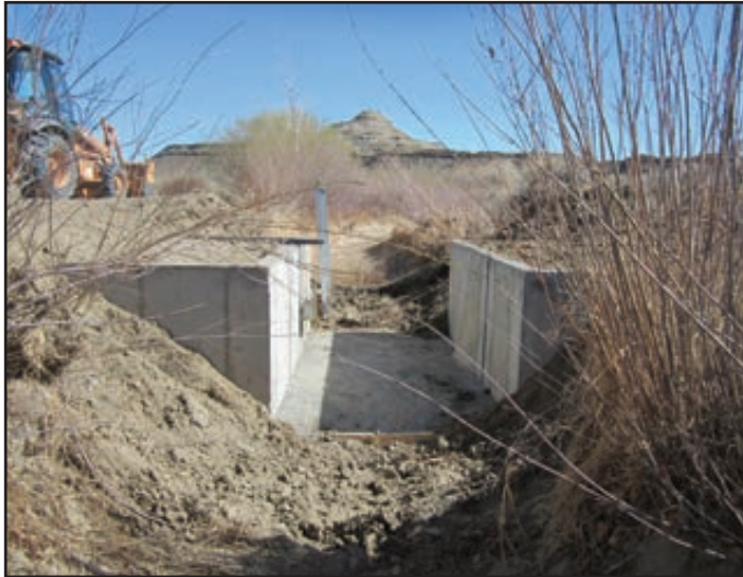
Figure 69. New concrete check in Big Fork canal at Yellowtail WHMA.
