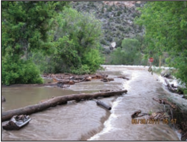
Figure 62. Tensleep Creek flooding and debris jams prior to the road washing out on June 30, 2011.
