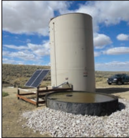
Figure 98. Well #2 windmill was replaced with solar power, stock tank and ~16,000 gallon storage capacity.
