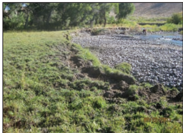
Figure 99. Looking upstream in 2011 at an eroded and trampled bank.
