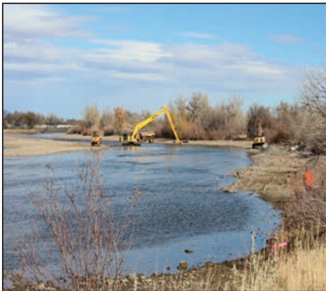
Figure 15. North Platte River restoration construction, October 2016.
