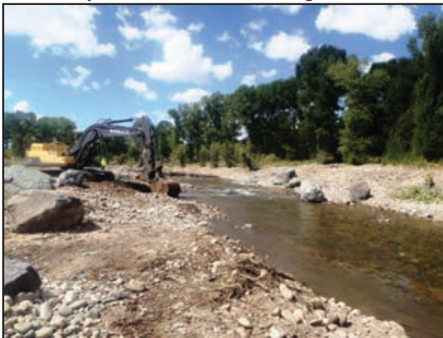
Figure 122. Reconstructing rock constructed riffle structure for the Encampment River - Boykin maintenance.
