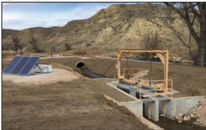
Figure 177. Dual vertical slot fish ladder (left) located between the Pratt and Ferris #1 dam and diversion ditch. Photo on right depicts a close-up view of the operating ladder.
