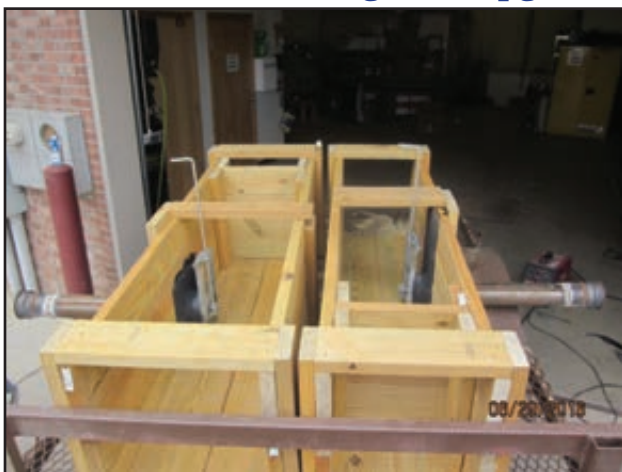
Figure 168. Bud Love WHMA irrigation system diversion boxes.
