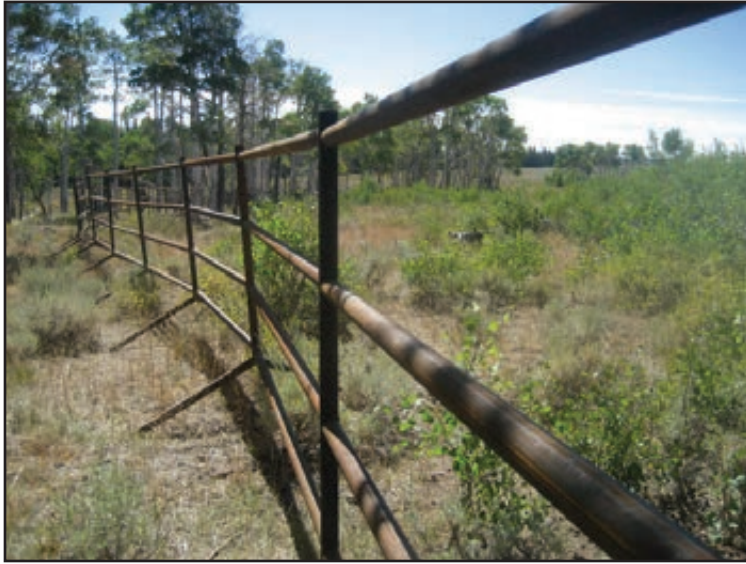
Figure 79. Portable steel jack fencing erected to protect young aspen trees from excessive browsing on Little Mountain.
