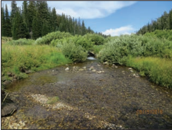
Figure 5. Before construction, perched outlet and scoured streambanks.
