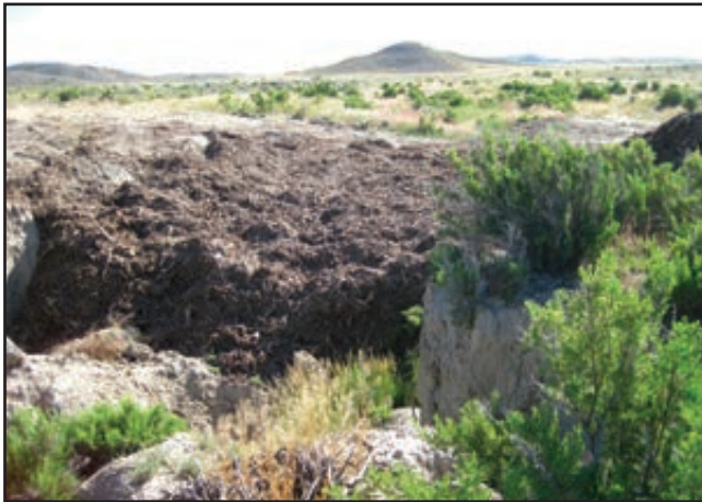
Figure 16. Shredded tree material placed in headcut.
