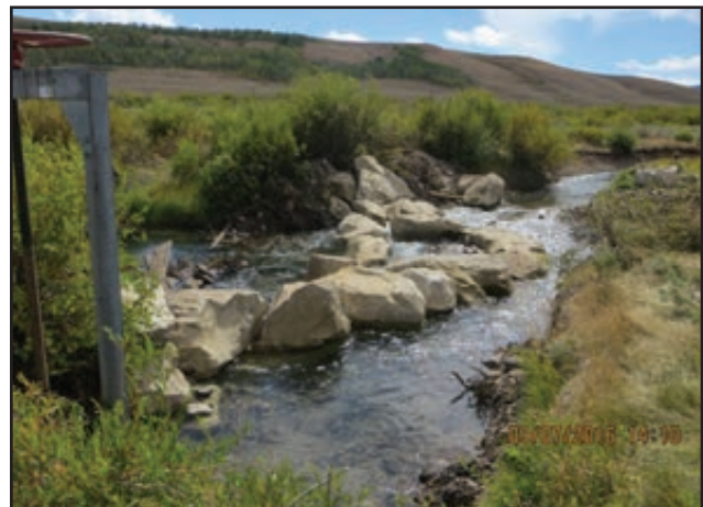
Figure 9. Fredell Ditch passage before and during construction; structure is 75% complete.
