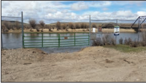
Figure 148. Newly installed gates and access parking improvements at Sommers Boat Launch PAA.
