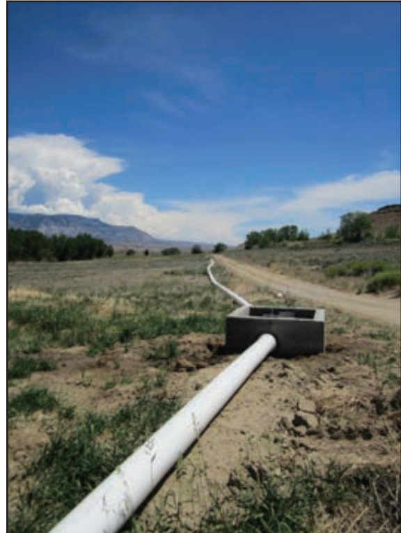
Figure 70. New diversion box used to split irrigation water on a permanent cover field.
