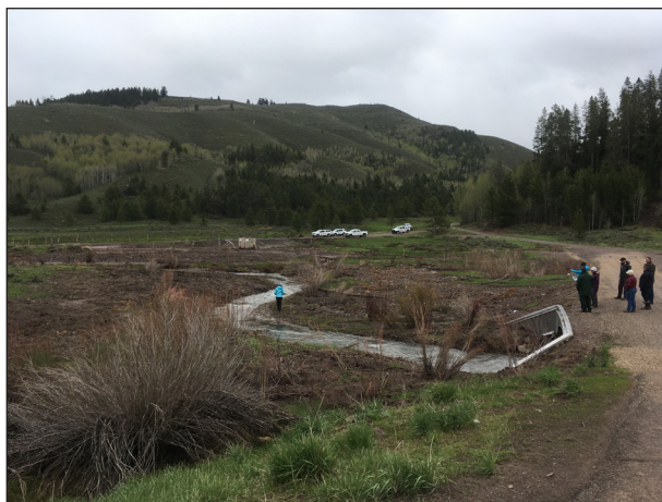
Figure 127. Partners tour the newly installed aluminum box culvert over Salt Creek.
