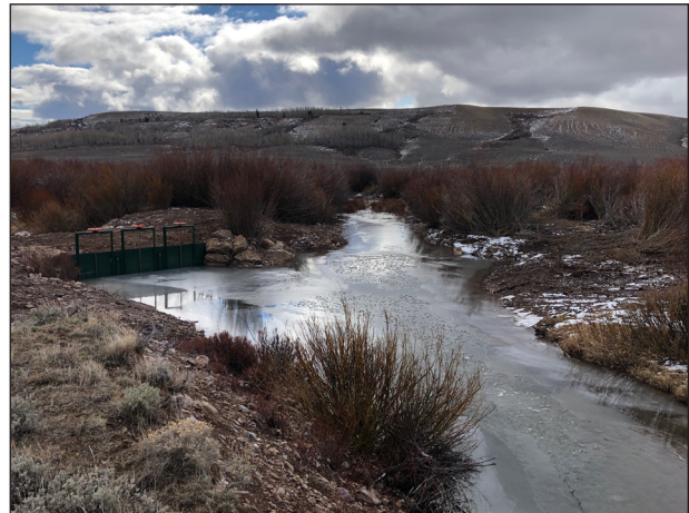
Figure 118. Looking downstream at new headgates and reactivated channel.
