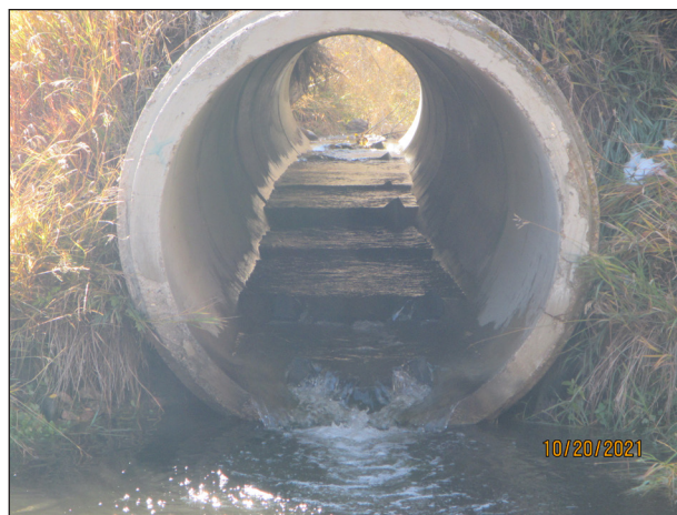
Figure 98. After baffle installation.
