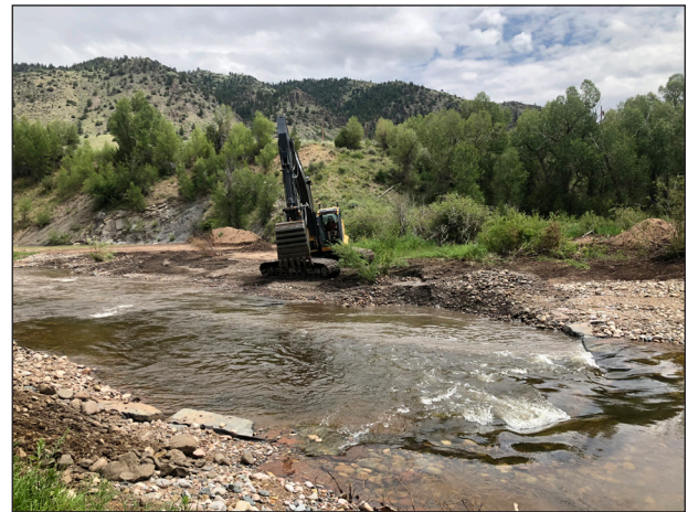
Figure 100. Laramie River - Jelm Restoration channel grading.
