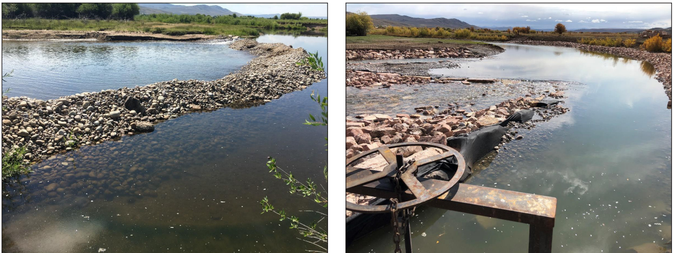
Figure 42. Morris Brothers Diversion before (left) and after (right) construction.
