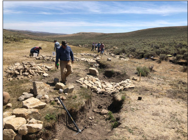
Figure 130. Volunteers installing Zeedyk structures.
