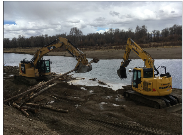
Figure 122. Dueling excavators at the New Fork Gas Wells Restoration.
