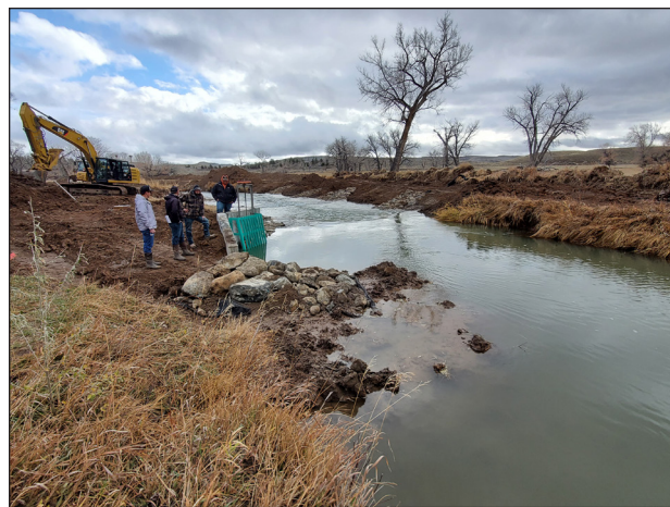
Figure 146. Renovation of the Moffett Diversion on the Middle Powder River.
