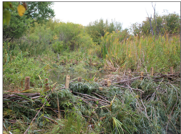
Figure 139. BDA structures along Amsden Creek.
