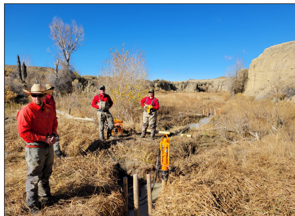
Figure 3. The crew finishing the last post on a Bolton Creek BDA installation.
