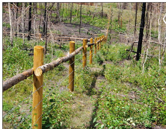
Figure 110 Pole top fence constructed post-wildfire in high wildlife crossing areas.
