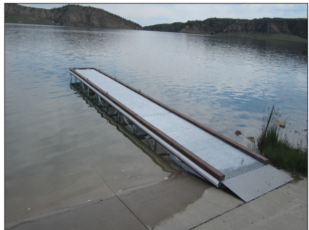
Figure 39. Boat dock installed at Upper Sunshine Reservoir.
