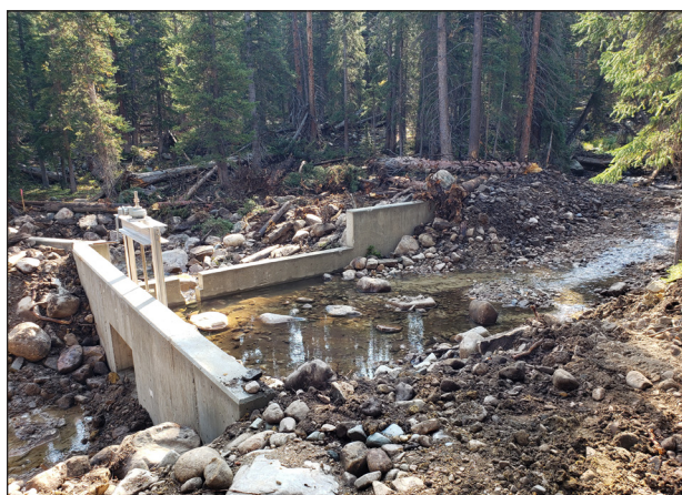
Figure 89. Carlson creek diversion.
