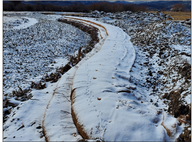
Figure 50. Flat Creek pool and toewood construction November 2021.
