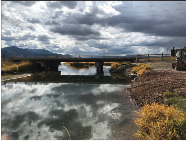
Figure 57. PAA maintenance on Salt River.
