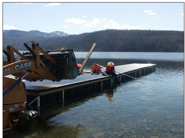
Figure 117. Installing new dock at New Fork Lake.
