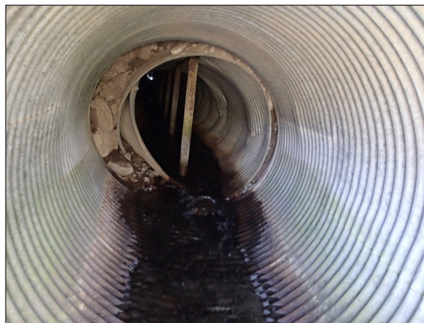
Figure 21. Oliver Gulch HWY 296 culvert is supported by multiple metal beams.
