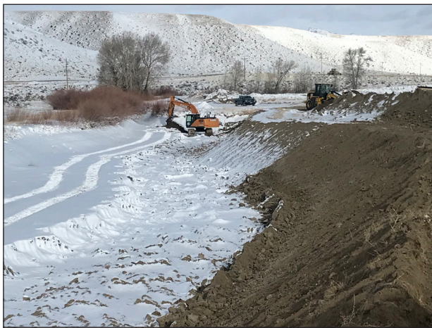
Figure 77. Settling pond maintenance on Spence Moriarty WMA.
