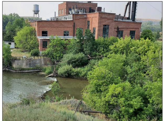
Figure 158. Cooling water intake structure.
