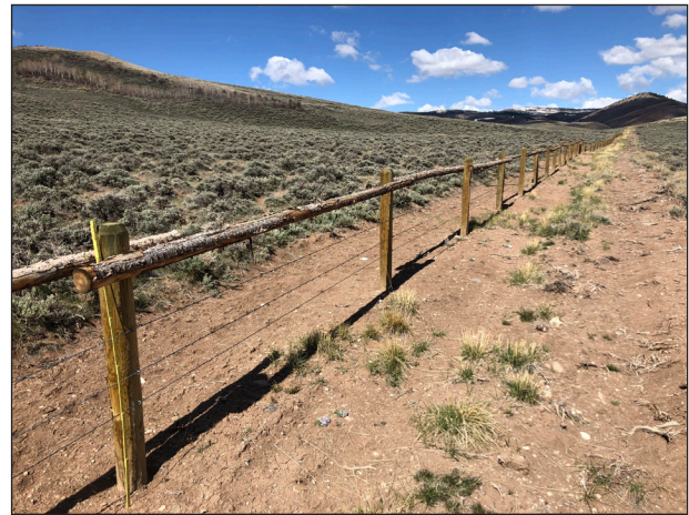
Figure 120. Completed top-rail wildlife friendly fence.
