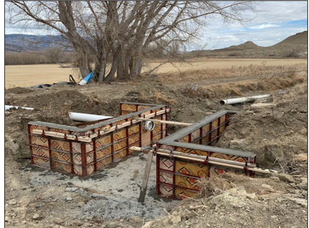
Figure 32. New concrete check for irrigation on Yellowtail WHMA.
