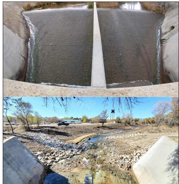
Figure 143. Before and after channel grade on Clear Creek upstream of Interstate-25.
