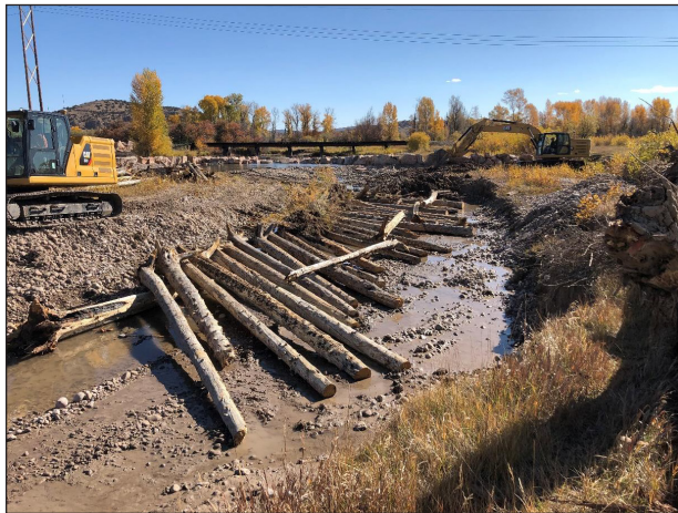
Figure 41. Toewood being installed downstream of Jon Sims Ditch.
