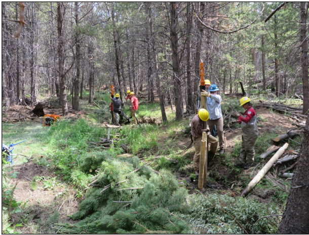
Figure 70. Installation of BDA's on Mill Creek.
