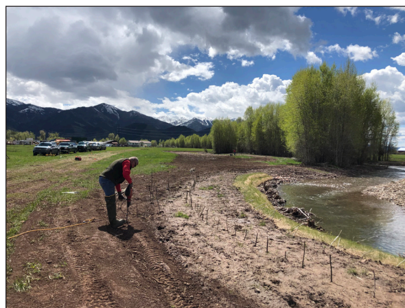
Figure 60. Planting willow poles on Swift Creek using a power drill.
