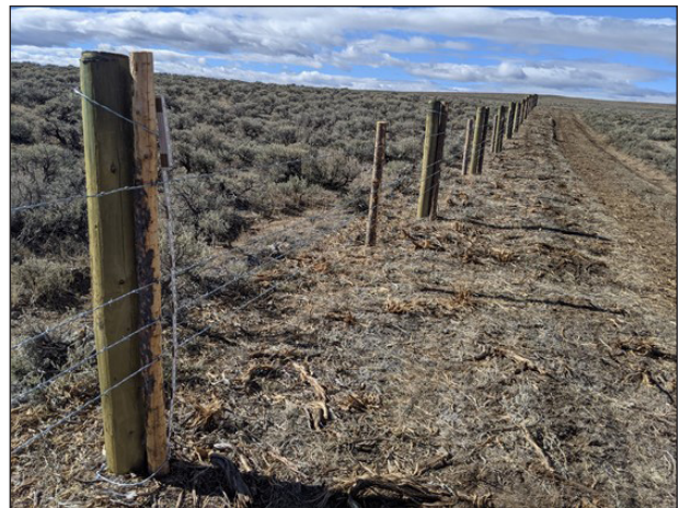
Figure 125. Completed fence on Mountain King Ranch.
