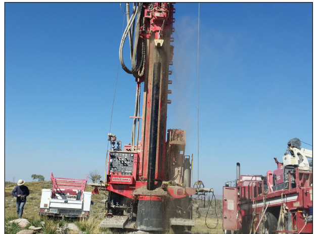
Figure 116. Well Drilling at Fall Creek WHMA.
