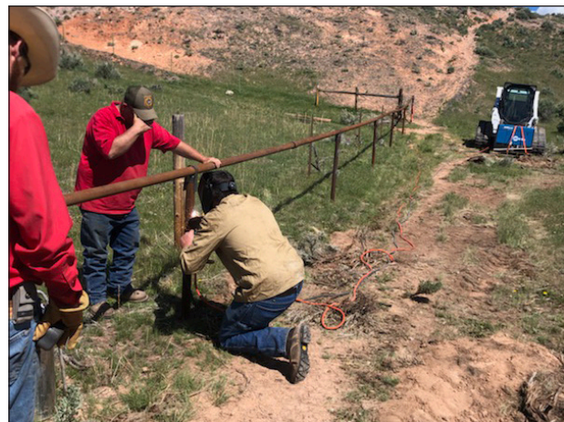
Figure 18. Installing new exclosure fence.
