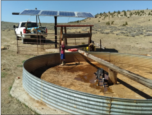
Figure 11. Installation of solar array pump at existing Baird well site.
