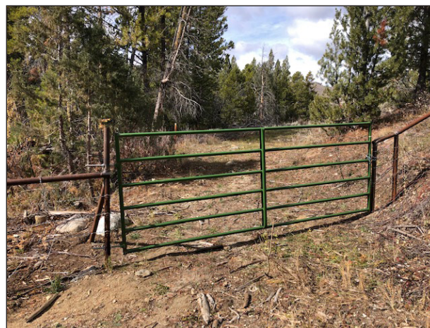
Figure 124. Gate install, Half Moon WHMA boundary fence.
